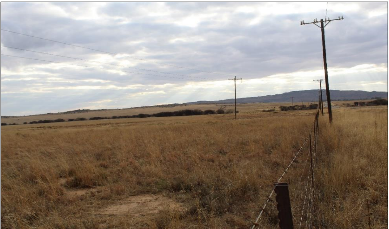
Figure 4. View of the powerline route with the hill which forms the western backdrop of Smithfield in the background
