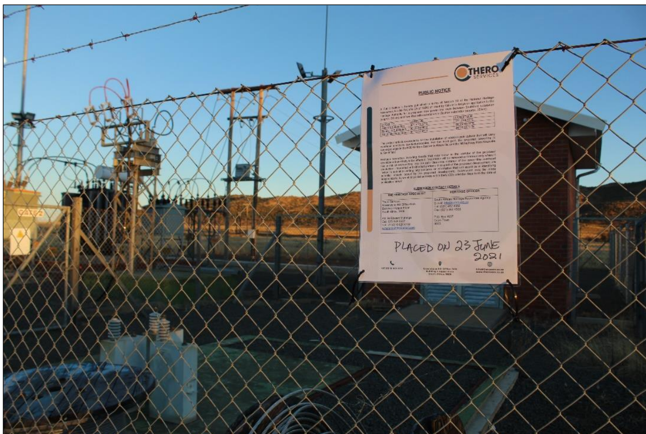
Figure 17: Public notice placed at the Eskom substation at Smithfield
