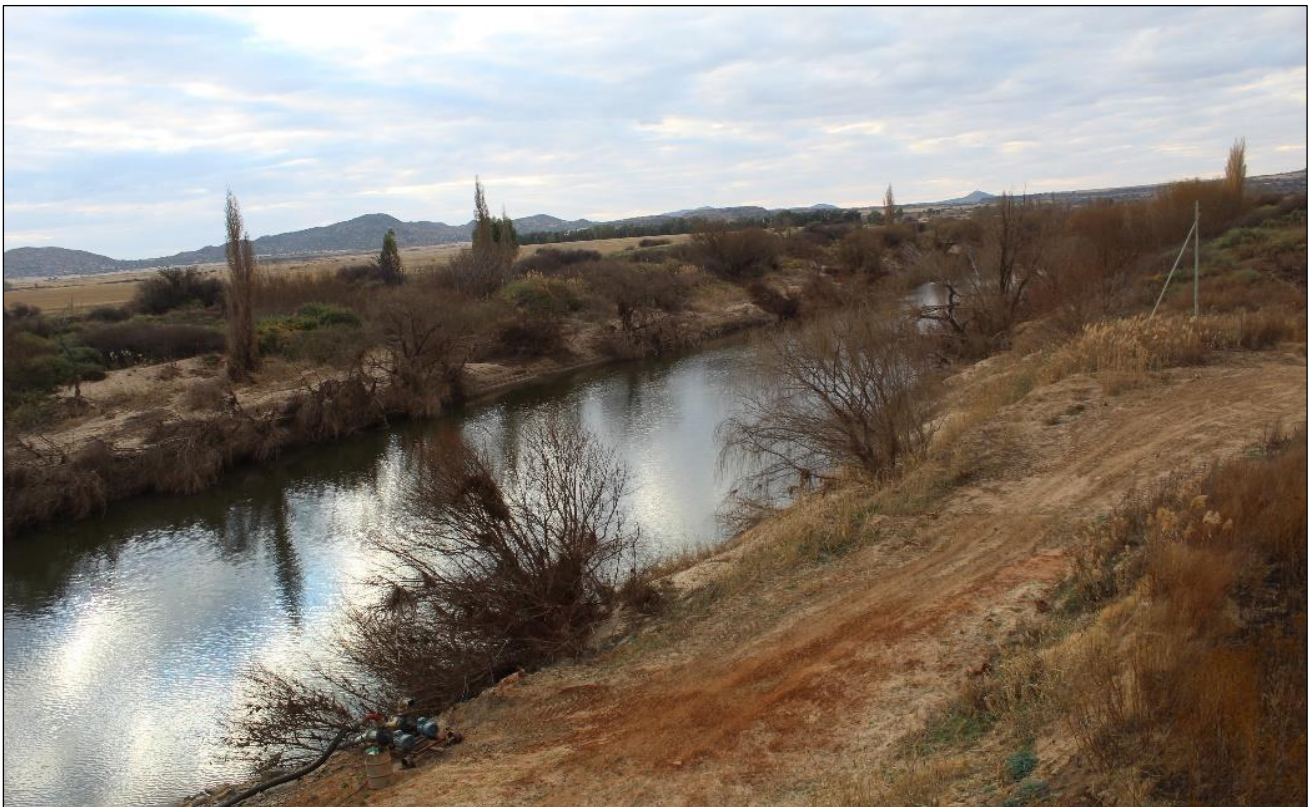
Figure 6: Powerline will cross the Caledon River on the north side of the Caledon River Bridge
