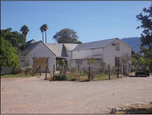
Figure 35: The rear of the parsonage.
