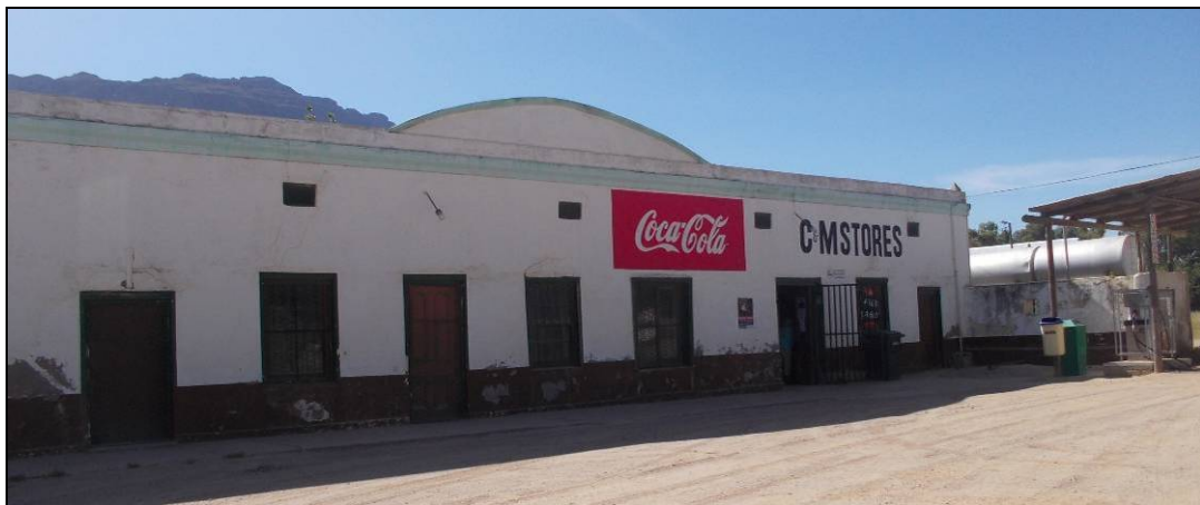
Figure 37: A commercial store in an art deco style.
