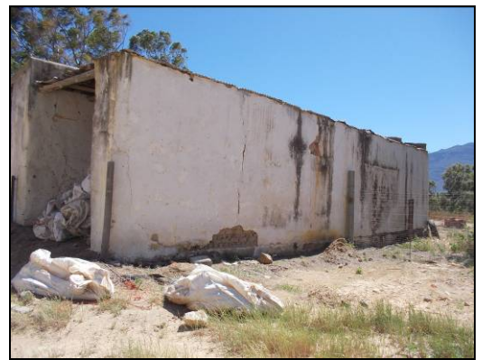
Figure 29: The south side of the outbuilding at Kleinberg.
