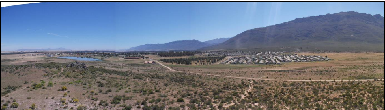
Figure 46: View towards the northeast from the rocky ridge south of Saron. The historic core of the village lies among the many trees, while the newer township developments are to the south (right and side in this image) and west (barely visible behind the dam in picture).
