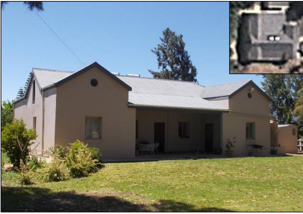
Figure 30: The main house at Die Mond. The inset shows the roof plan with the front at the bottom.
