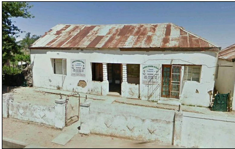
Figure 39: An early 20 th century or possibly late 19 th century house with later modifications.
