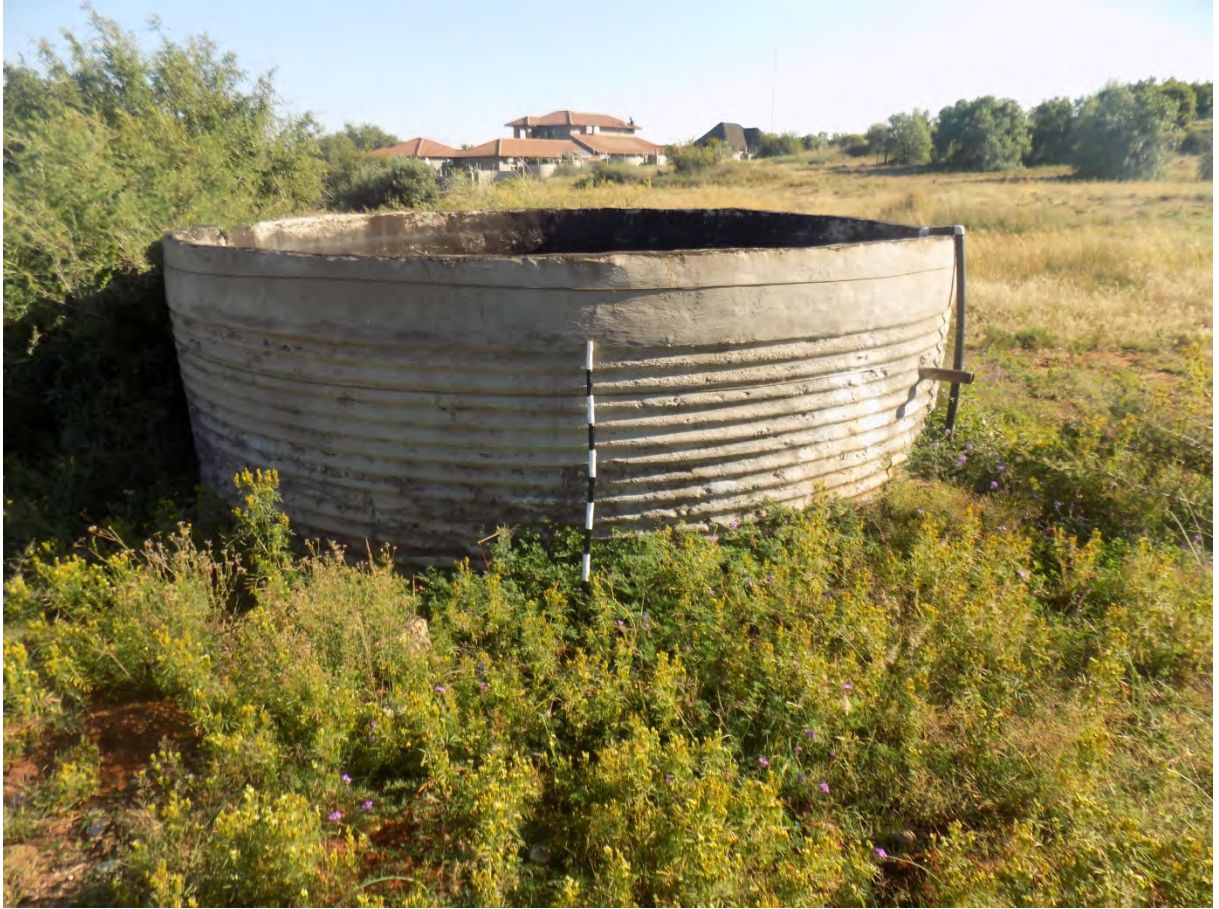
Figure 9. Modern dam, still in use.
