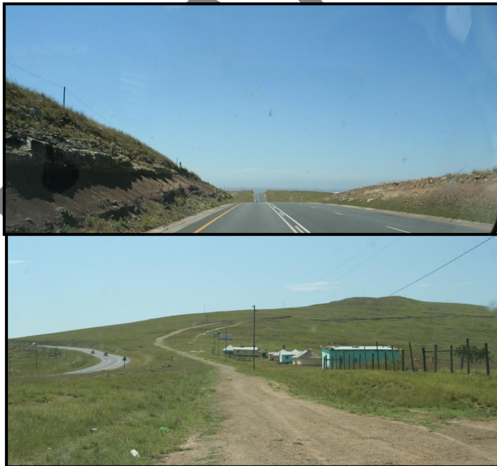
Fig 7: General Road View
