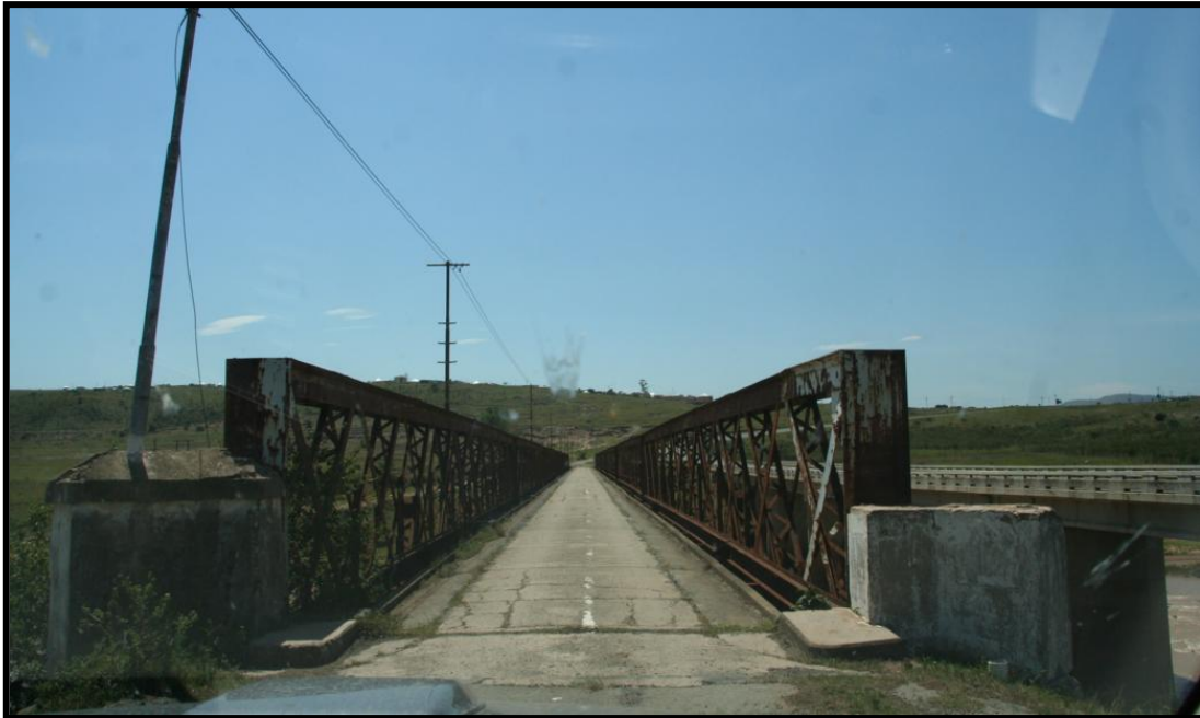
Fig. 16: Original Bashee River Bridge
