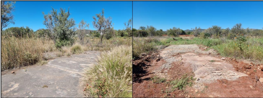
Figure 8-5: View of a building floor and foundation structure in the project area at TWRD-FT01.
