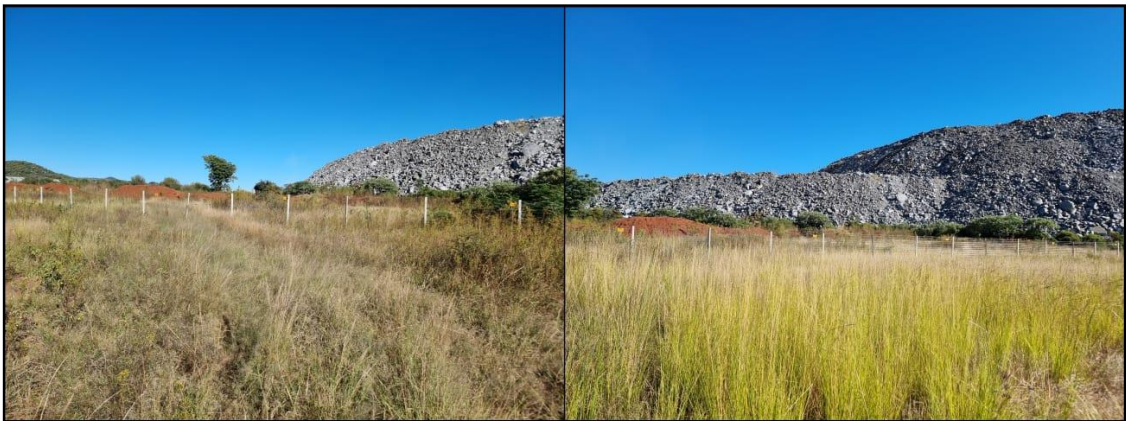
Figure 5-6: View existing WRD along the northern and western borders of the project area.
