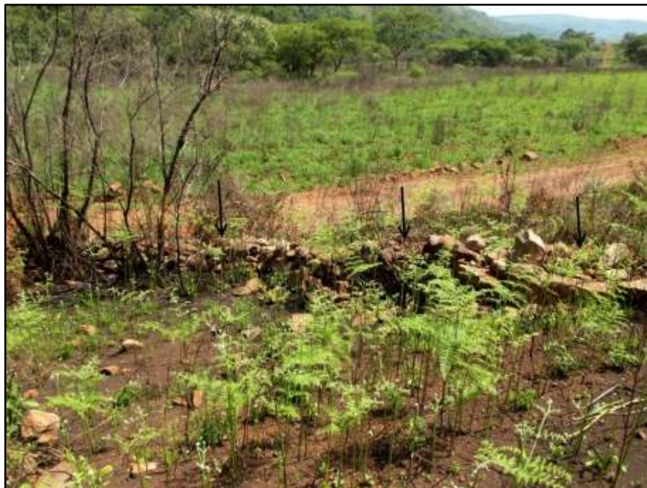
Figure 6. Site BL 4A. The collapsed oval-shaped wall viewed in a north-western direction.
