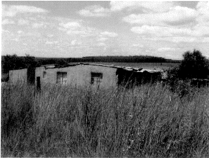
Figure 7: Some of the existing houses at Jabulani
