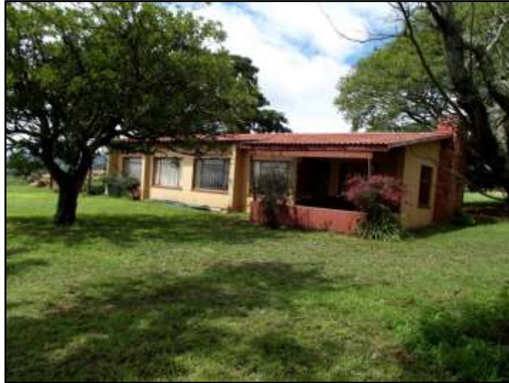
Fig. 1. Site TRB 1. The farmstead. Photo taken in a southern direction.
