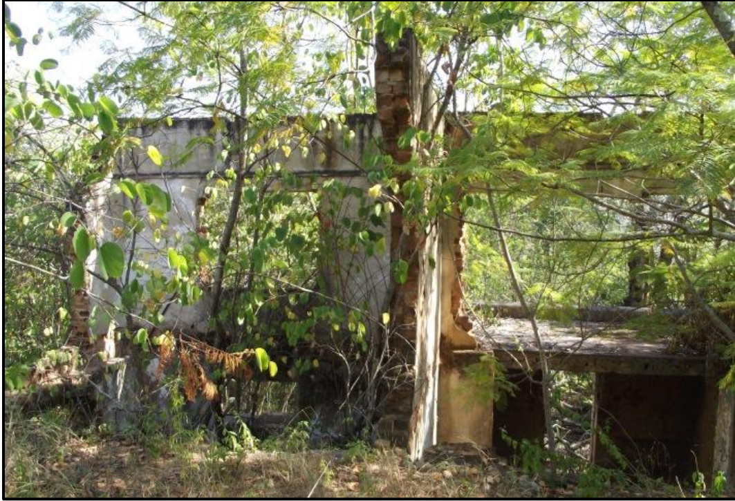
Fig. 3. Site NTR 3. The ruined remains of a large double storey house.
