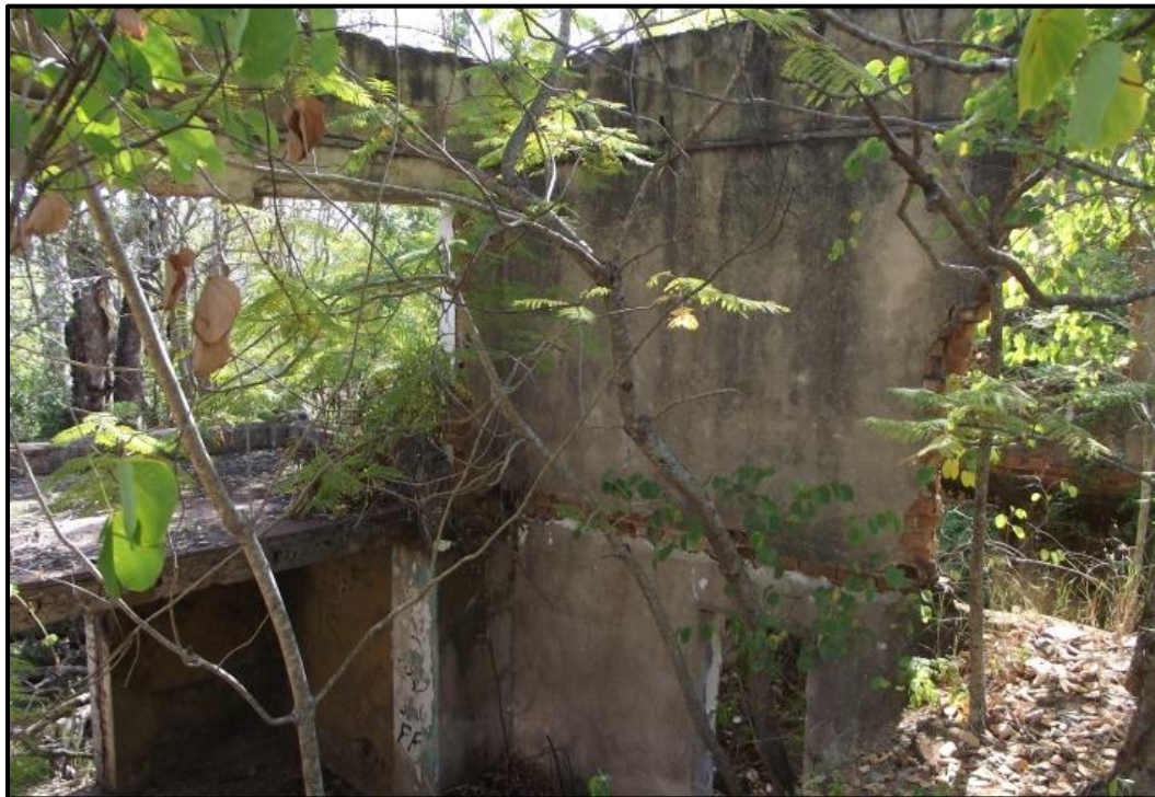
Fig. 4. Site NTR 3. The remaining walls, view in a south-western direction.
