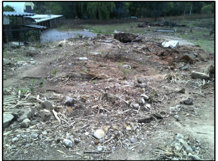
Figure 5. Demolished remains of house.
