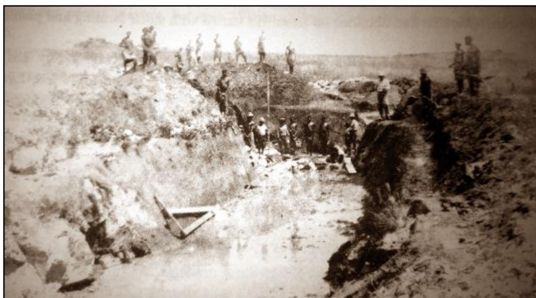
Fig. 4.2. Early settlers constructing an 25km water canal from the White River to irrigate their farms (taken from Bornman, 2015).
