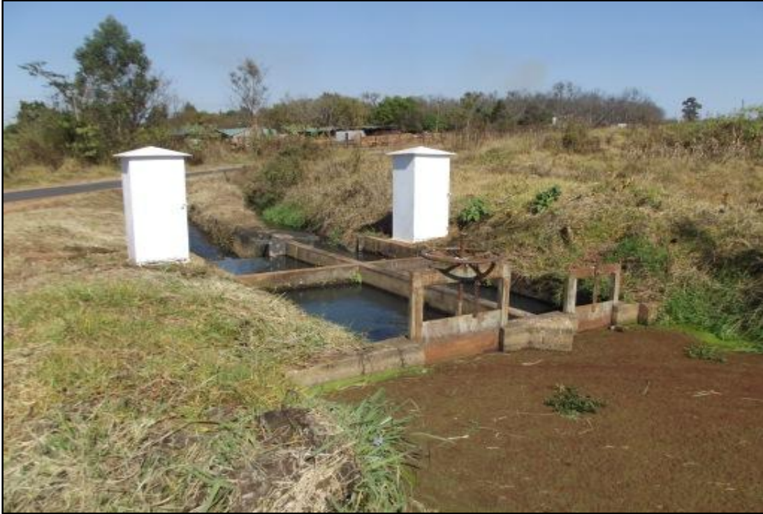
Fig. 13. Site WWA 12. A section of the historic water canal. Photo taken in southern direction.
