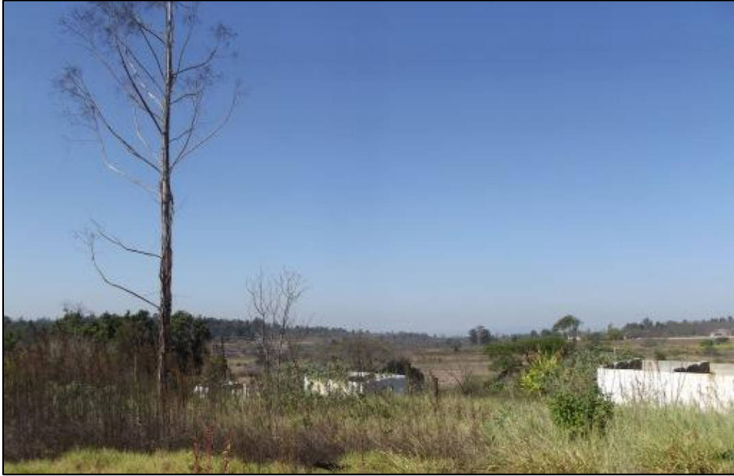
Fig. 11. Site WWA 4. Three of the old farm workers dwellings, they also have been vandalised and roof, doors and window frames removed. . Photo taken in south-eastern direction.
