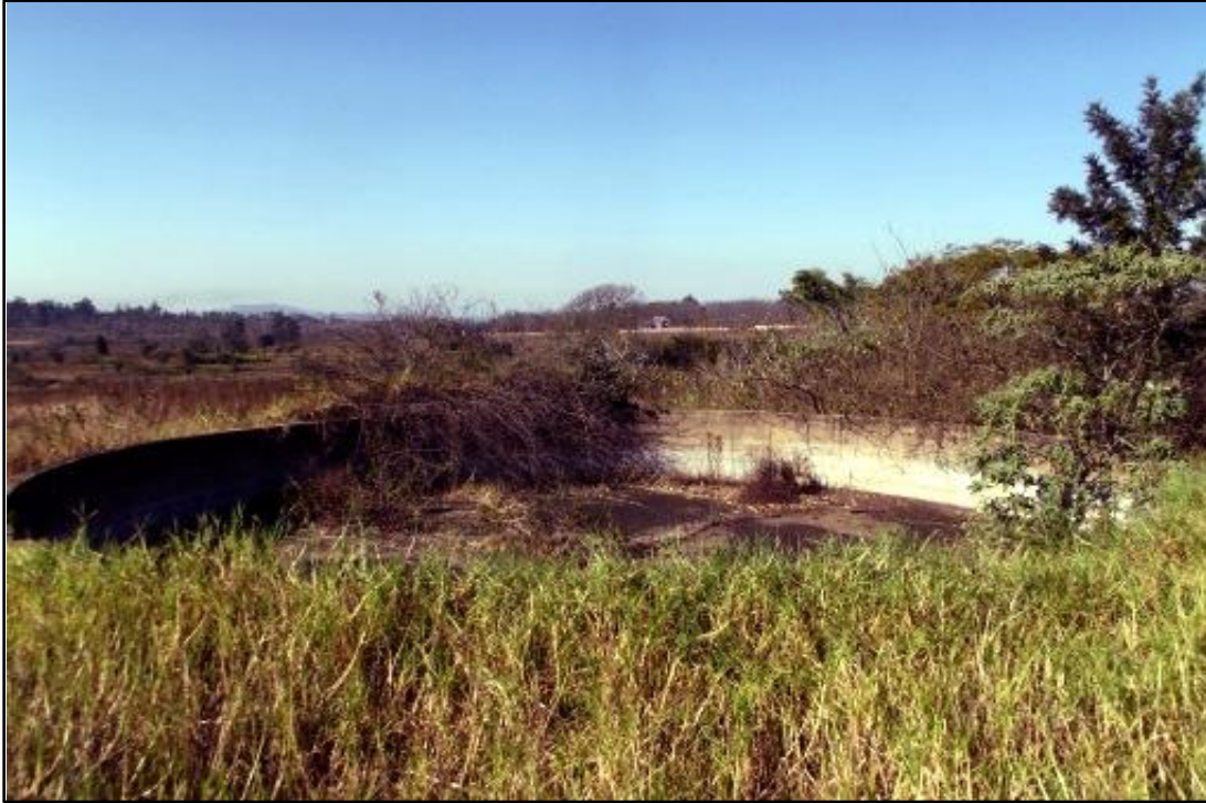
Fig. 3. Site WWA 2. An old concrete dam, possibly for irrigation or household water.
