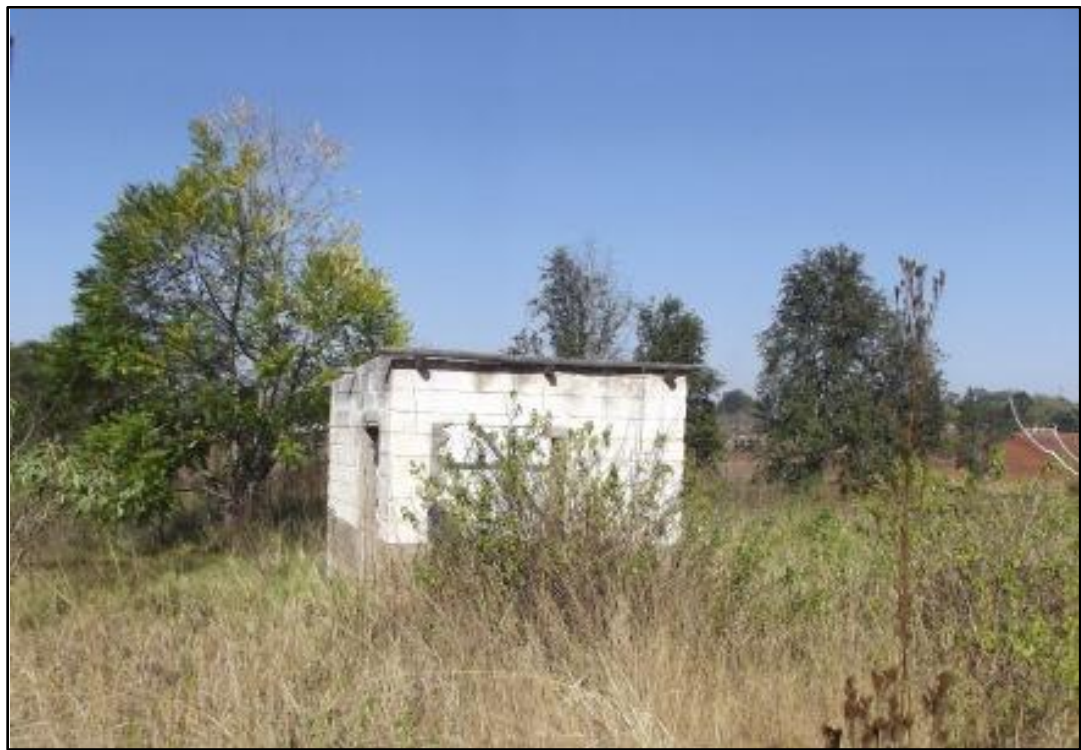
Fig. 6. Site WWA 3. Associated outbuilding. Photo taken in southern direction.
