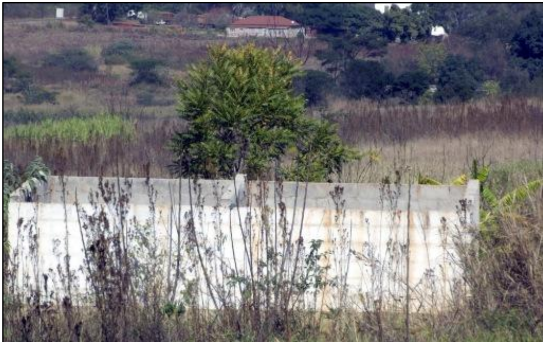
Fig. 12. Site WWA 4. Old farm worker's house, close-up photo of the ruin. Photo taken in southern direction.
