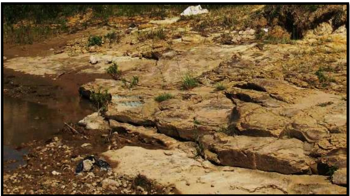
Figure 13. L1526: position for Culvert 1.
