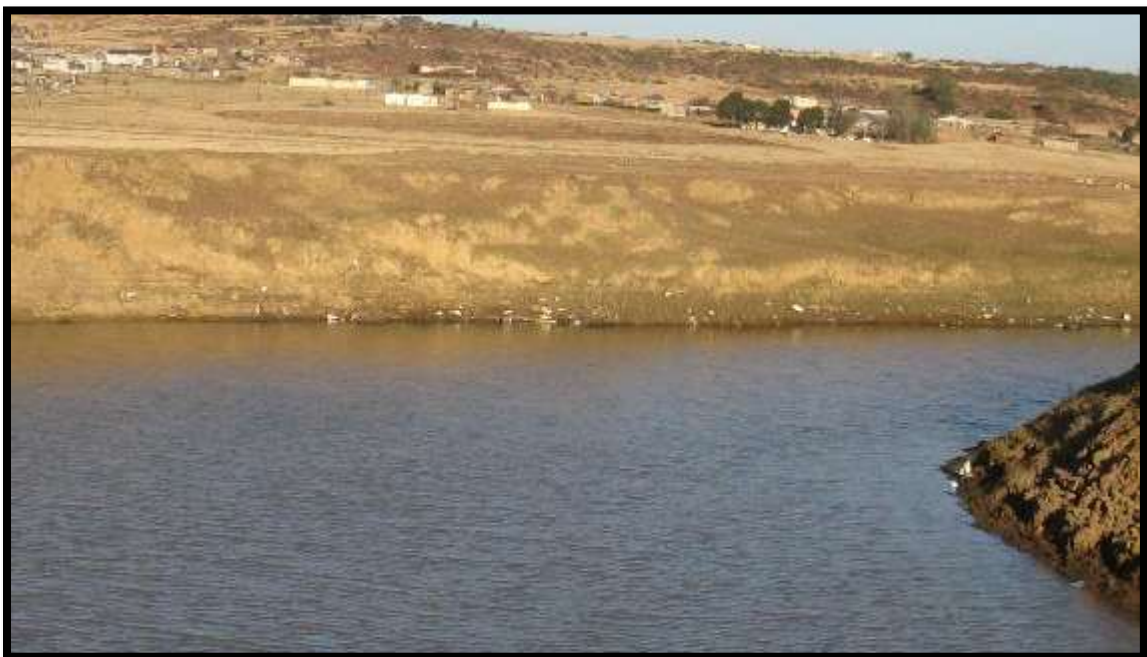
Figure 9. Woodstock Dam, a well known landmark, is situated to the immediate west of the project area.
