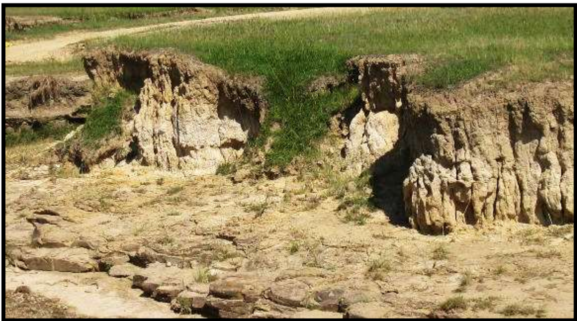
Figure 11. District road L1511 leading to river crossing for proposed culvert.
