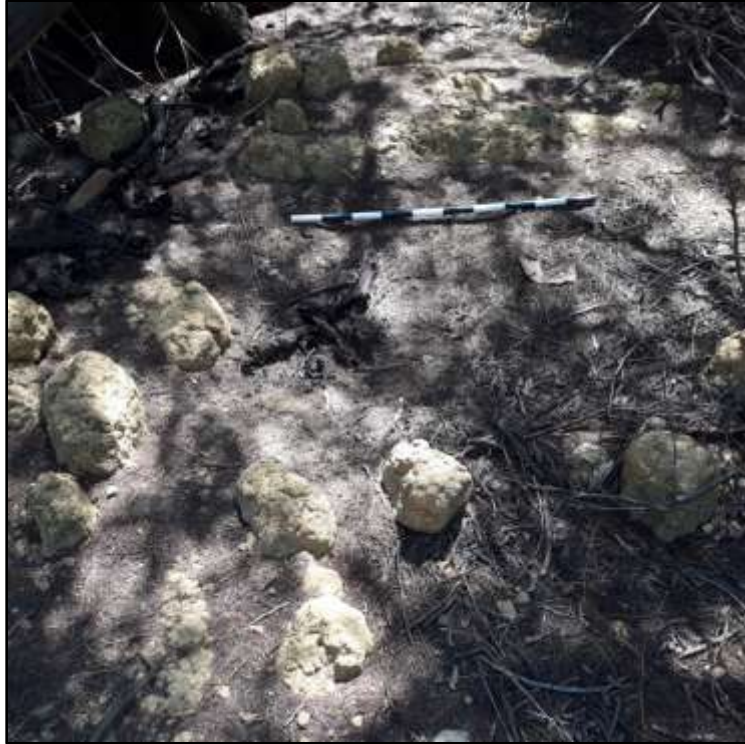
Fig. 5. Site TRP 3. Collapsed walling and some remains of a foundation.
