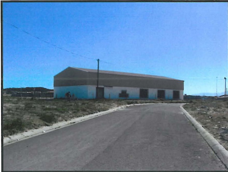
Fig: 4 Industrial building to the South West of the site.
