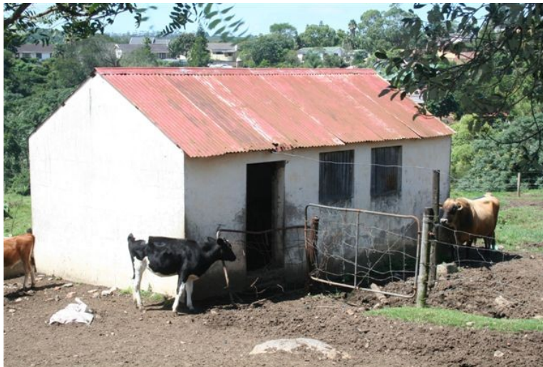
Fig 6: shed on Palm Valley farm
