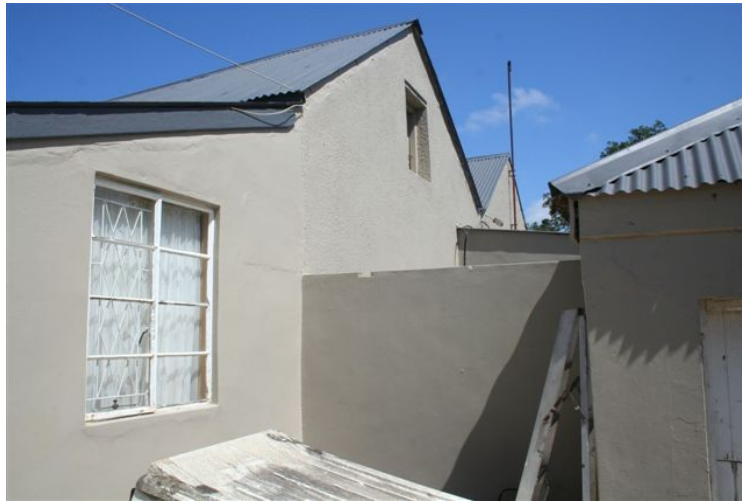
Fig 7: roof-space ventilator and M-roof form
