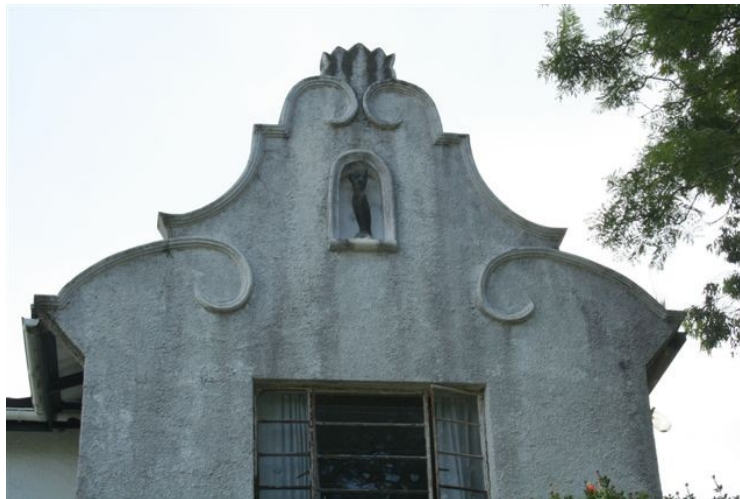
Fig 4: Close up of gable
