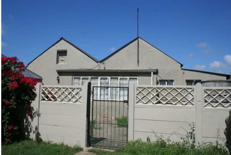
Fig 9: view of M-roof form with valley gutter
