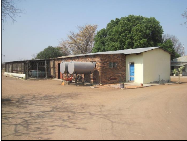
Figure 25: View of the garage/storeroom on the eastern side of the house.
