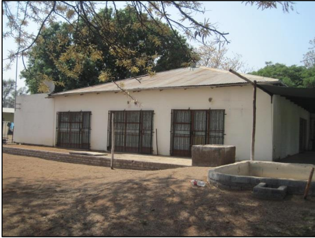
Figure 21: View of the old farmhouse from the north.
