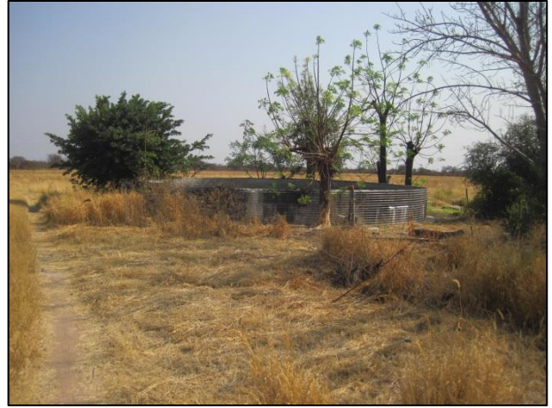
Figure 6: View of the corrugated dam on the site.
