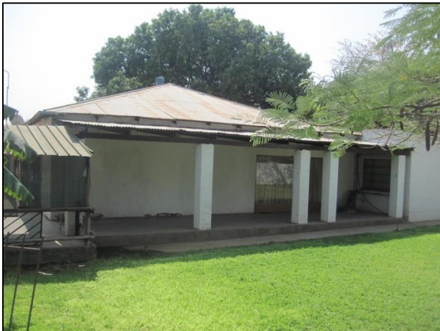
Figure 23: View of the veranda on the western side of the house.
