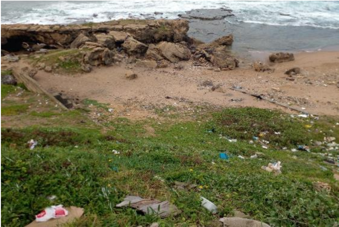
Figure 14: Area below outlet point of culvert
