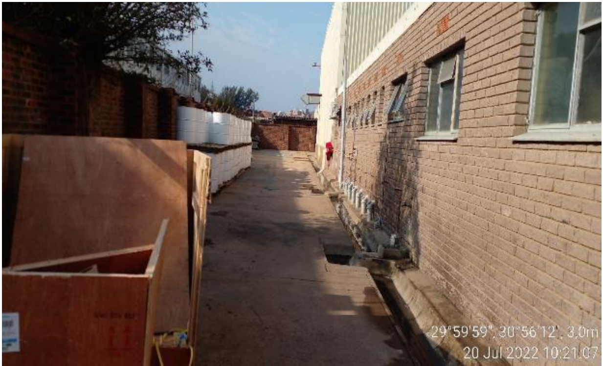
Figure 6: Boundary wall between businesses at Joyner Road start of culvert
