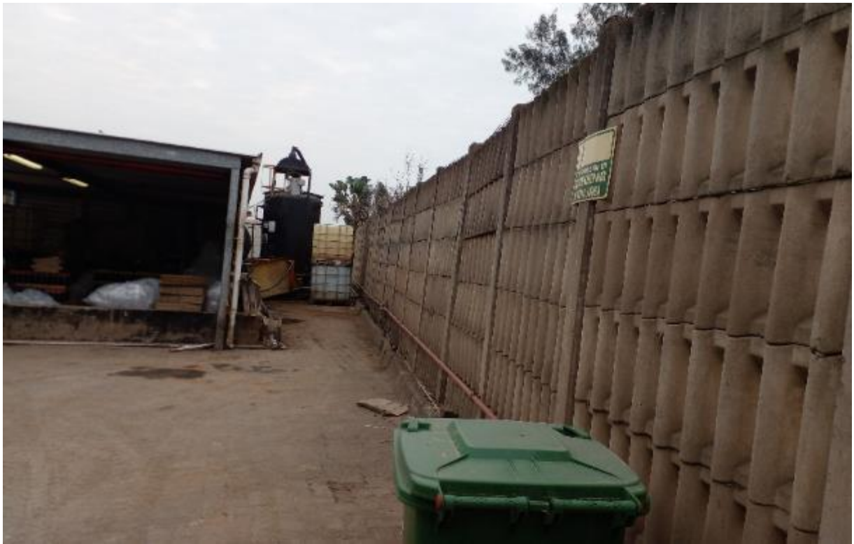
Figure 8: Machinery near route of culvert
