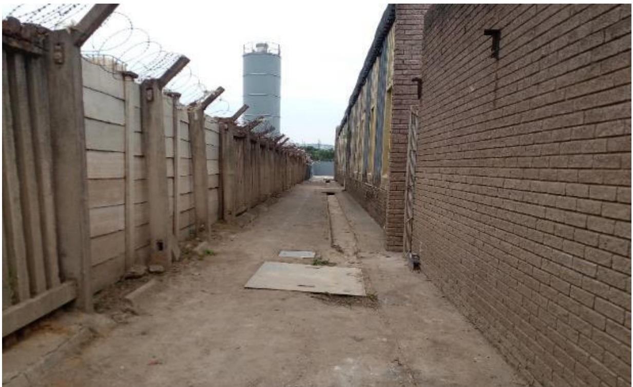
Figure 7: Culvert route 200m south-east of Figure 6
