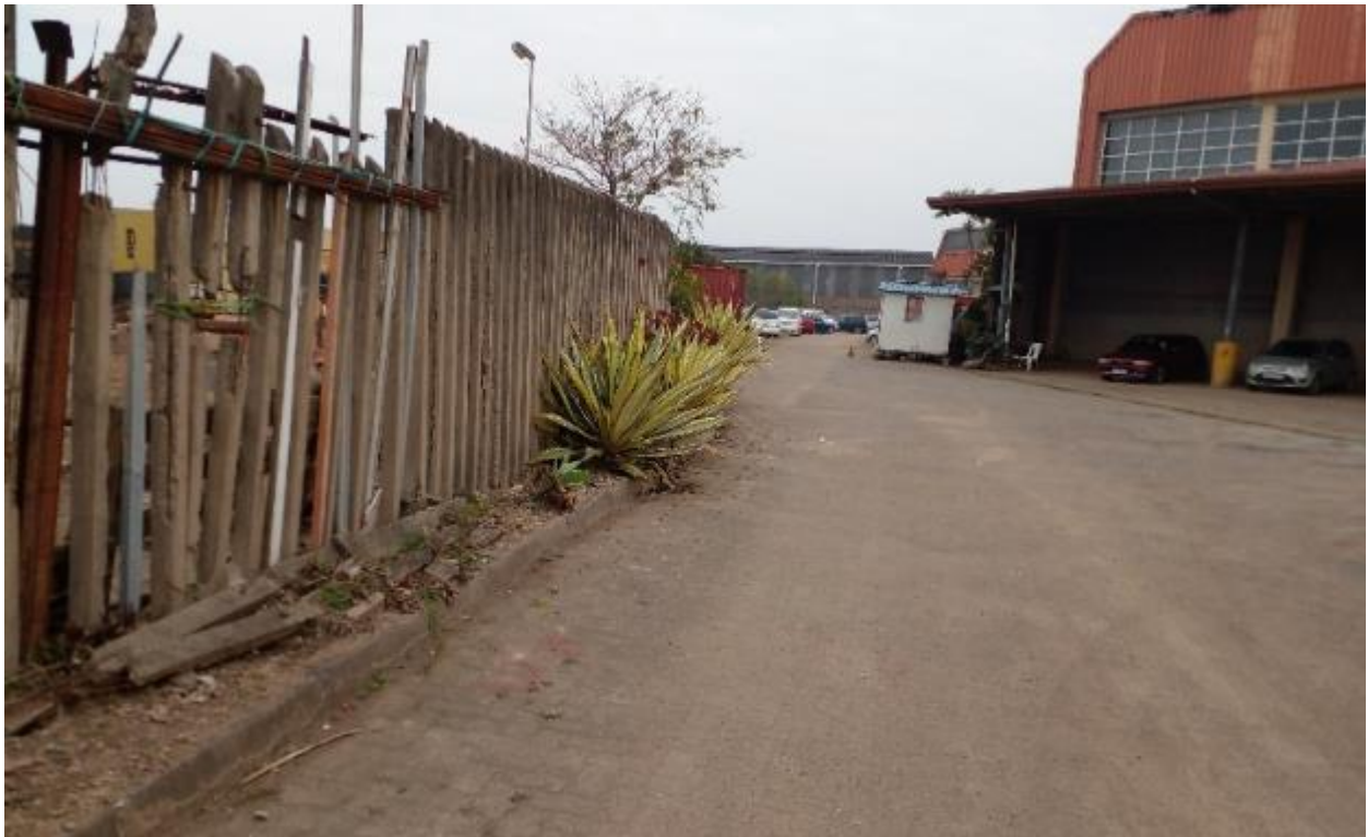
Figure 10: Culvert route on boundary of properties
