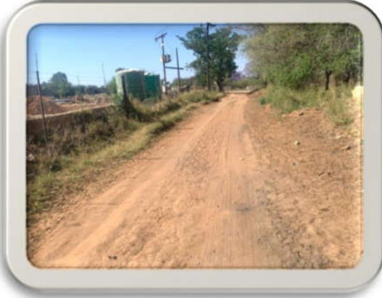
Gravel Road (Intersection B)
