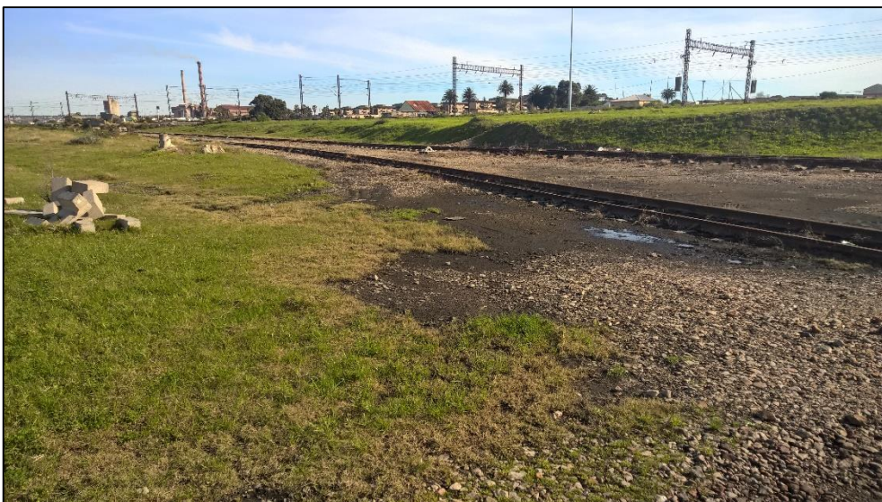
Figures 8-10. View of the western area for the proposed construction of the Transnet Security Wall showing the surface disturbances caused by the construction and maintenance of the main rail line and water dissuasion and retainer walls.
