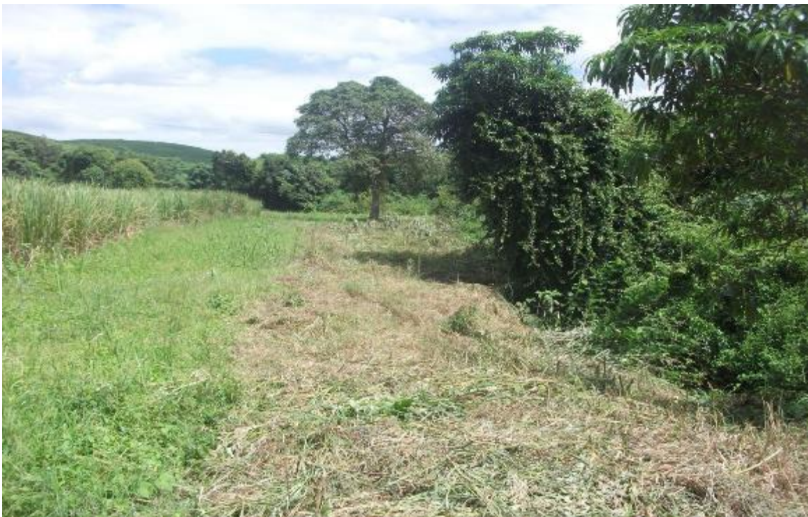
Figure 6: Clearing of area along Hlawe River
