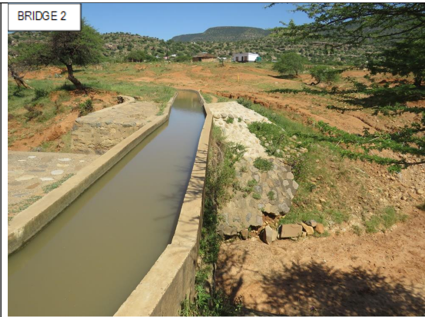
Figure 9: View of the modified /repaired canal
