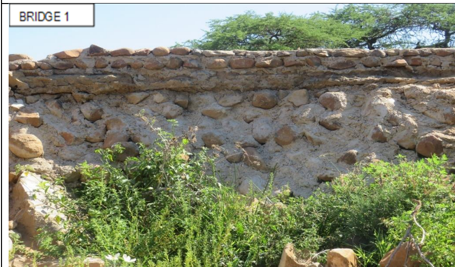
Figure 6: Stone masonry at bridge one
