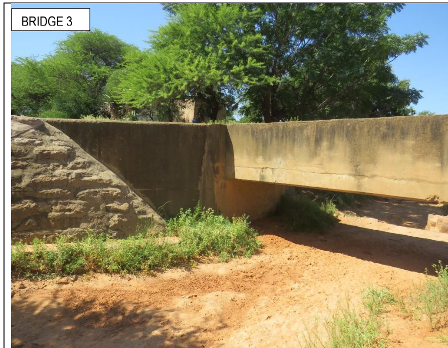
Figure 10: View of concrete bridge three
