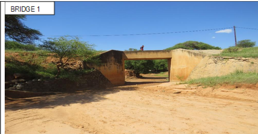
Figure 5: A view of bridge one from a distance
