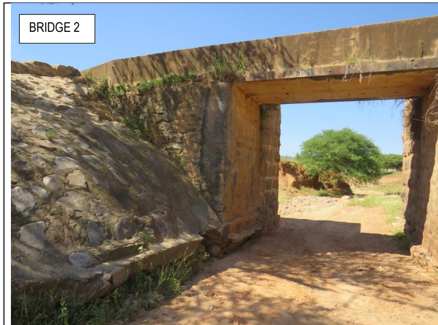
Figure 8: View of the concrete bridge two
