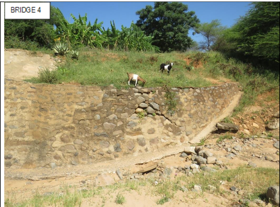
Figure 13: View of the surrounding environment at bridge four
