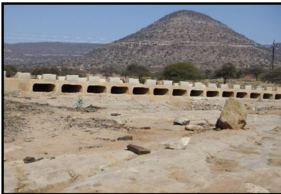
Figure 3. Photograph of water crossing at Twaleykhe Road.
