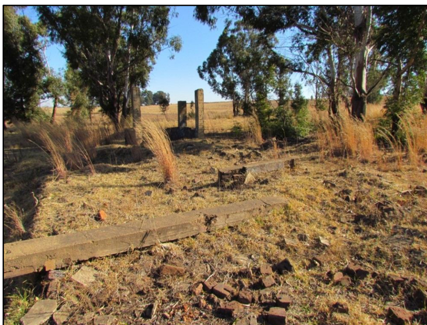
Figure 6-24: View from the south of remains of structure identified at H010
