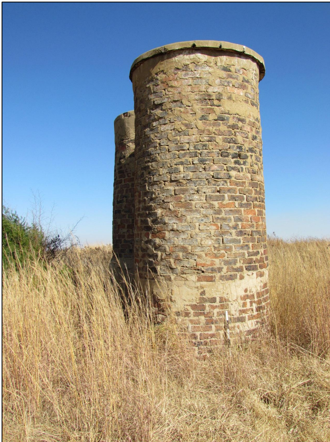
Figure 6-16: Cylindrical brick towers identified at H007
