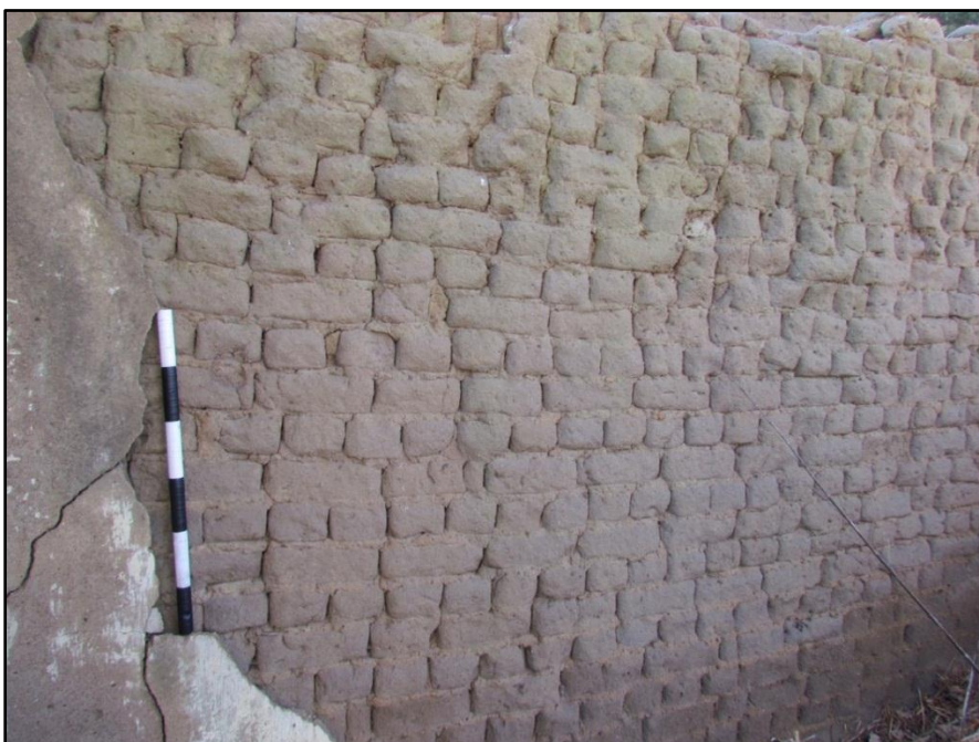
Figure 6-26: Mud brick interior walls of structure identified at H011
