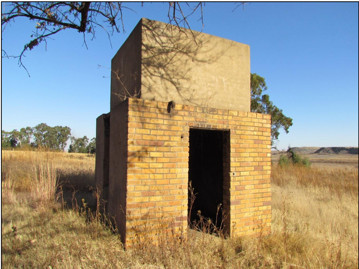
Figure 6-27: Water tower (water tank missing) identified at H011
