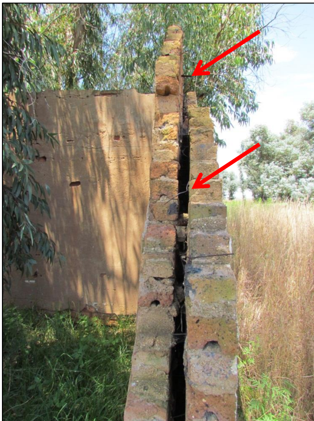
Figure 3-8: Close up of exterior cavity-wall at Site 2. Note metal wire reinforcing in the cavity.
