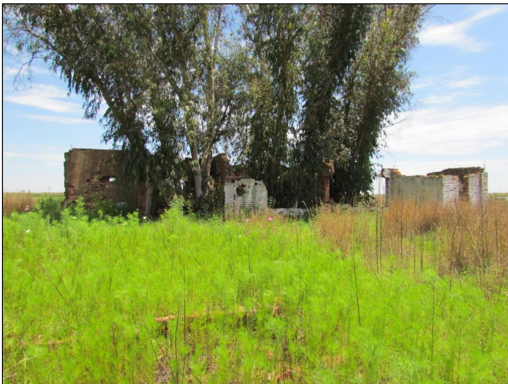
Figure 3-4: Eastern elevation of the main structure at Site 2
