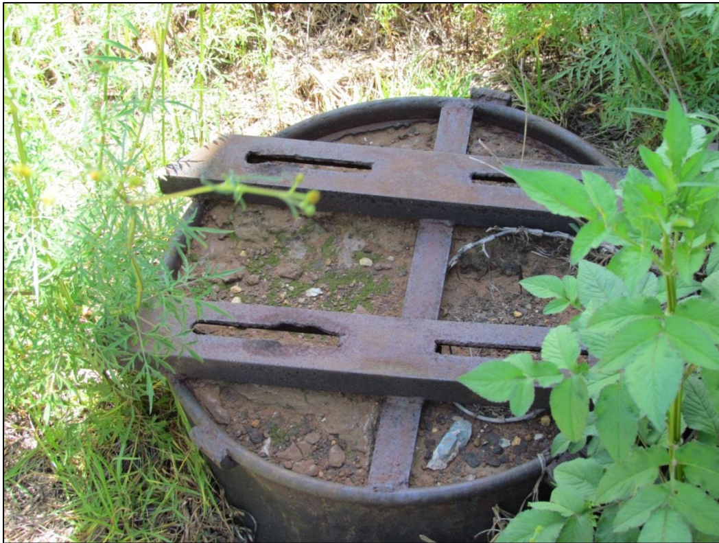
Figure 3-22: Borehole pump housing noted adjacent to water tower near borehole.
