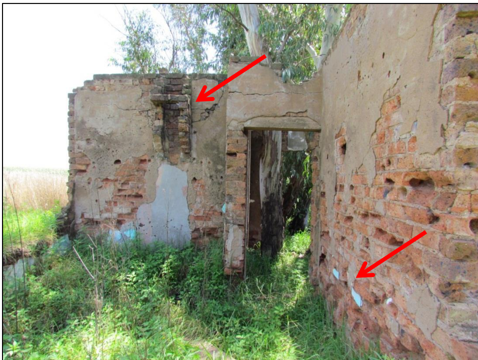
Figure 3-11: North Elevation of site 2 and view of kitchen area. Note remnants of kitchen chimney and light blue paint indicated by the red arrows
