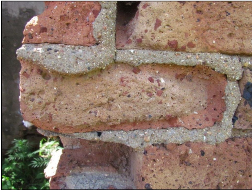
Figure 3-7: Close up view of fired bricks with cement and riversand mortar used in the construction of the main structure
