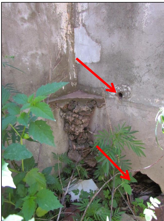
Figure 3-20: Interior view of the washroom with close up of bath support. Note the pipe inlet and outlet for the bath
