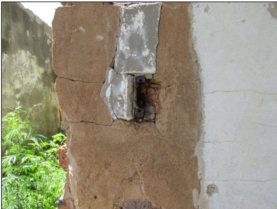
Figure 3-18: Remains of a switch on the eastern wall of the main bedroom at Site 2
