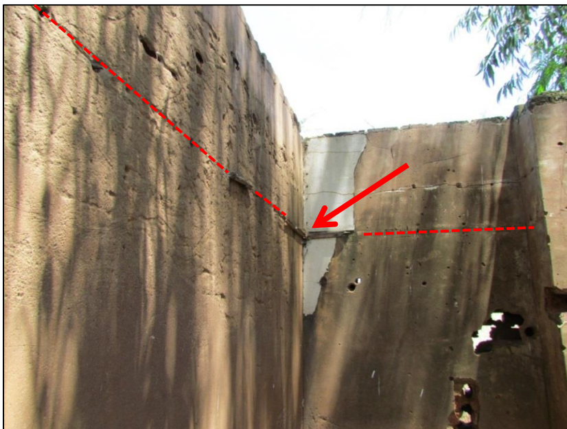
Figure 3-14: Section of wooden dado rail located approximately 2.5 meters above the floor level on the wall of the living room in Site 2
