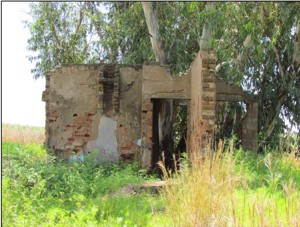
Figure 3-5: Southern elevation of the main structure at Site 2
