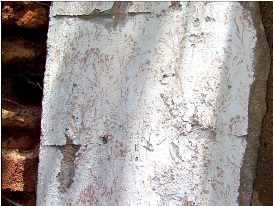
Figure 3-10: Close-up of wallpaper from entrance hall of Site 2
