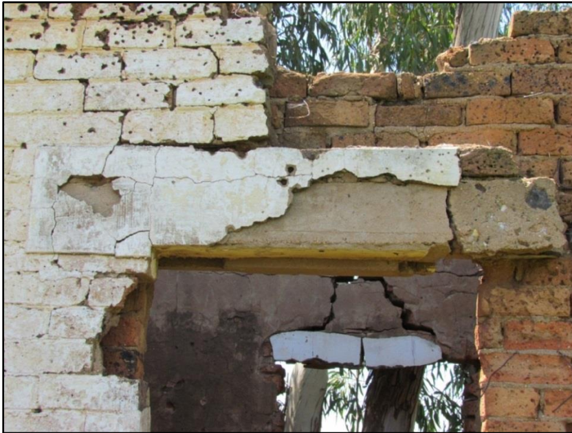
Figure 3-13: Window and door lintels in the small room adjacent the kitchen at Site 2
