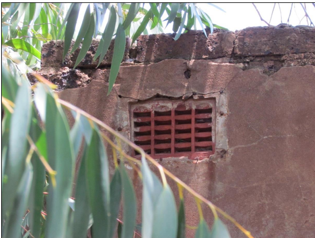
Figure 3-16: Air vent located at the top of a wall in the living room in Site 2
