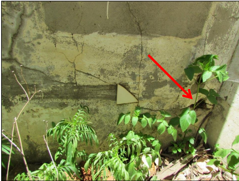
Figure 3-19: Interior view of washroom with fragment of white tile. Note pipe outlets for sink
