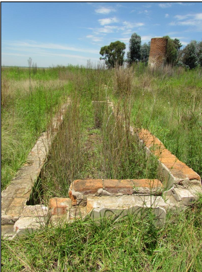
Figure 3-25: Brick water trough
