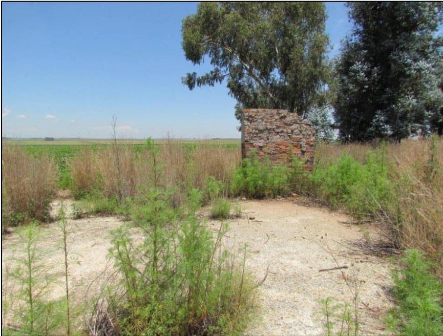
Figure 3-26: Large concrete floors located south-east of the main structure at Site 2
