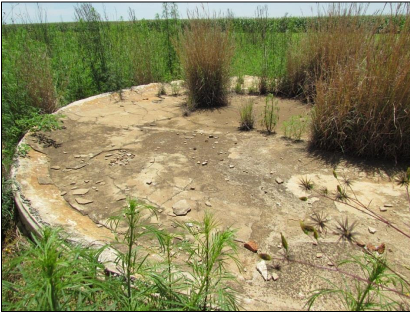
Figure 3-24: Reservoir foundation located next to water tower at Site 2
