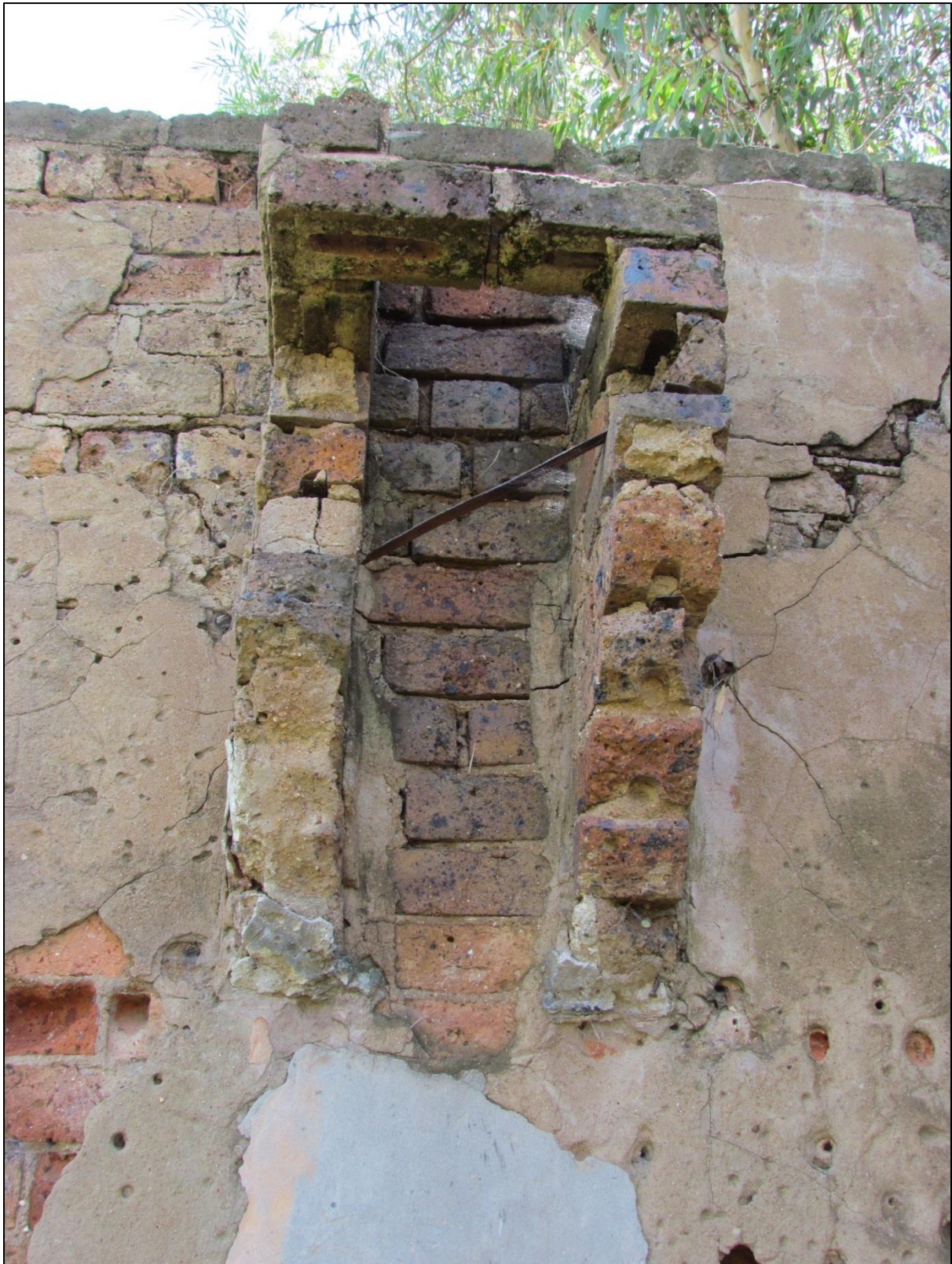
Figure 3-12: Close-up of kitchen chimney with metal flat-bar reinforcing visible
