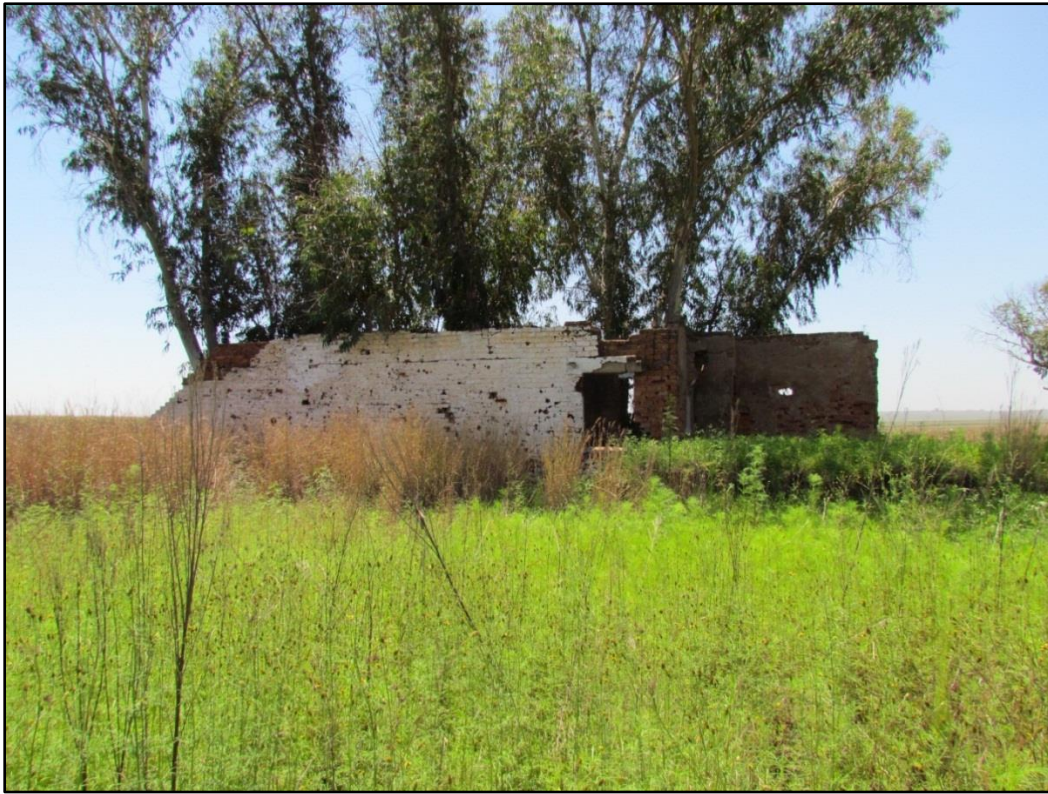
Figure 3-3: Western elevation of the main structure at Site 2
