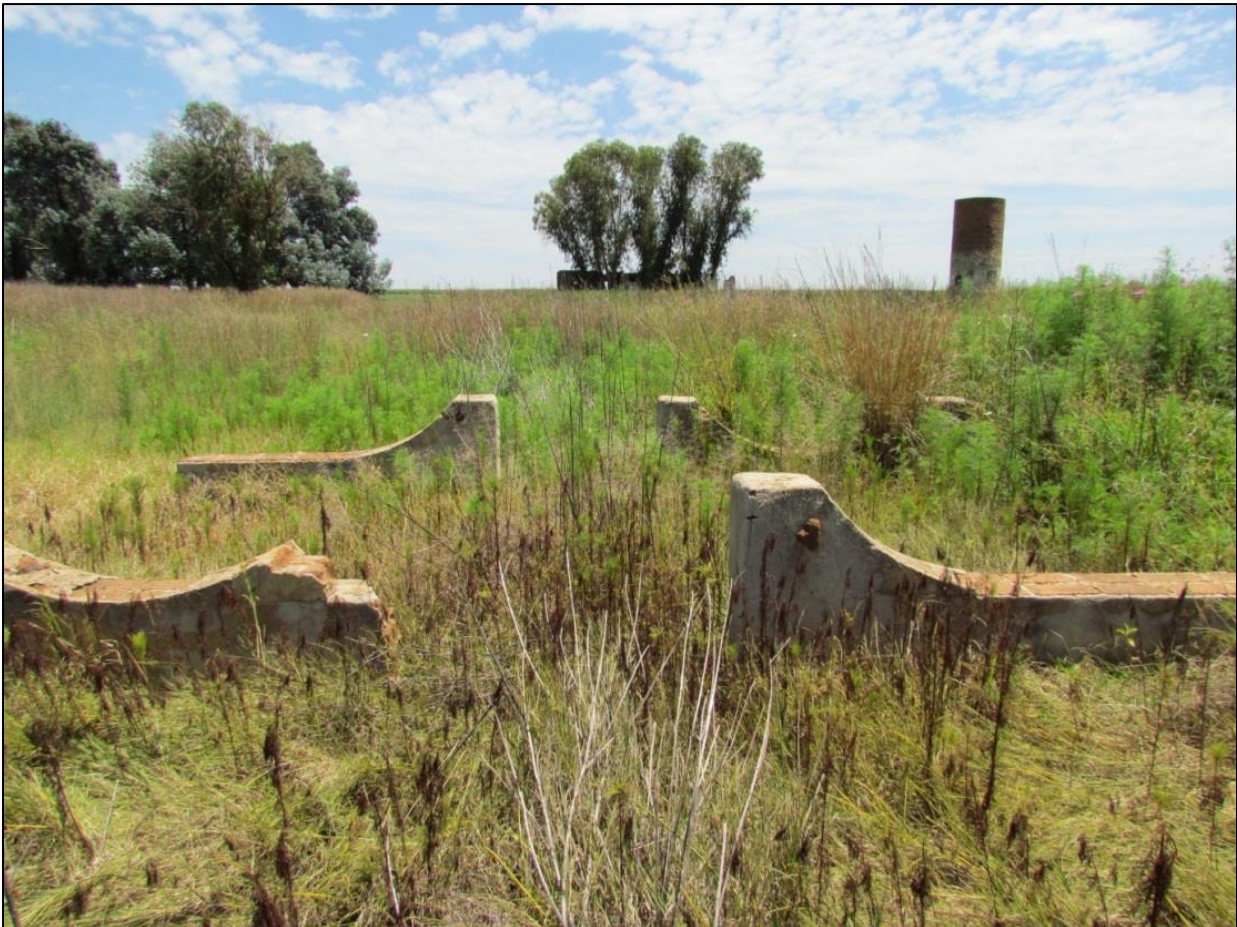
Figure 3-2: Eastern elevation of the main structure. Note the entrance gate and water tower
