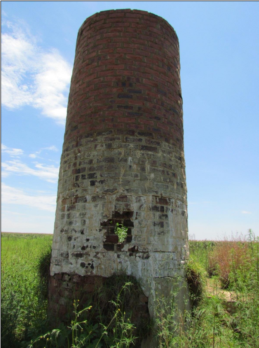
Figure 3-21: Brick water tower located north-east of main structure at Site 2
