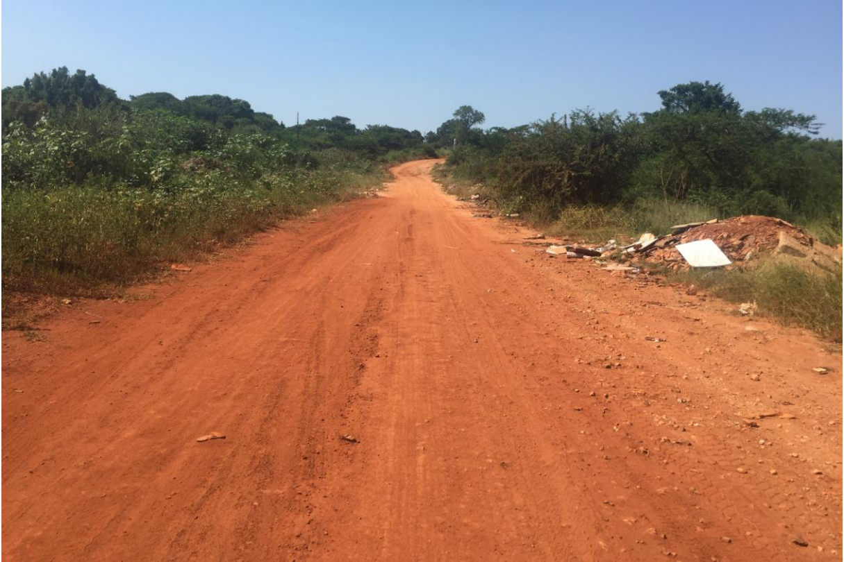
Figure 3: View of the southern section of the proposed area for construction.
