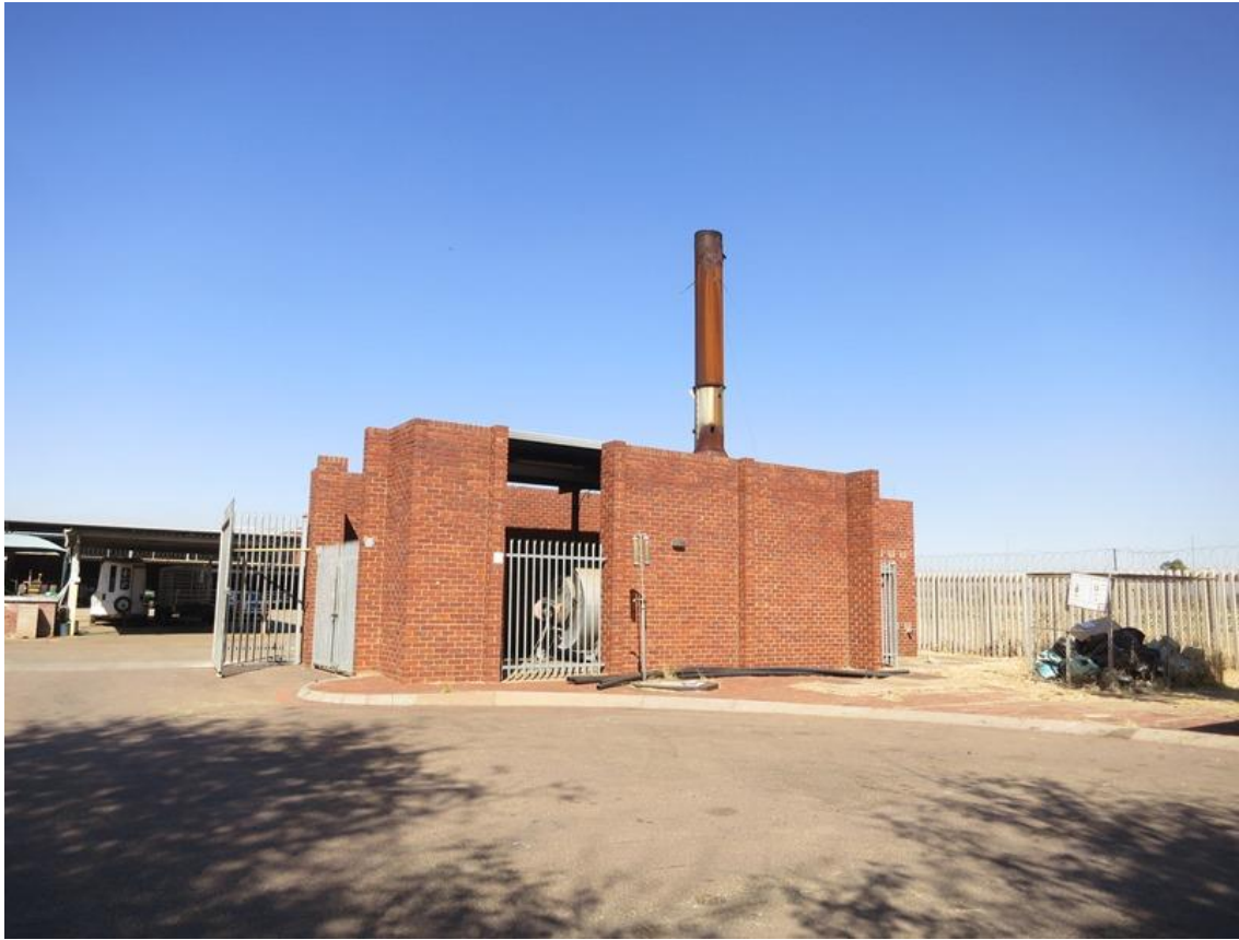
Figure 3: View of the Incinerator site and building.
