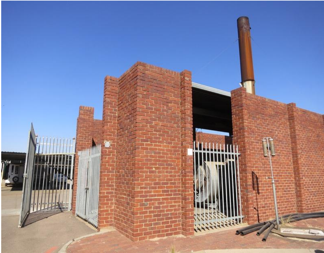
Figure 5: Closer view of the Incinerator and the structure housing it.
