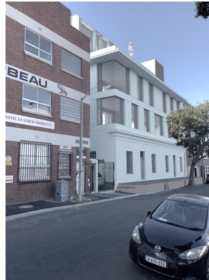
Views from no. 218 and no. 212 on Buitengracht
