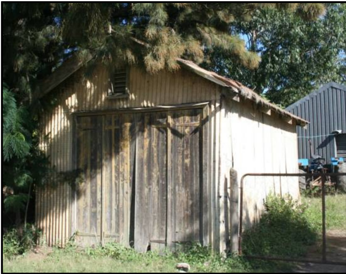
FIG. 13: BUILDINGS AT GAZ011
