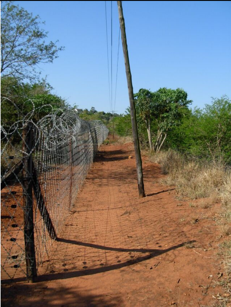
• Figure 9: General view of site
