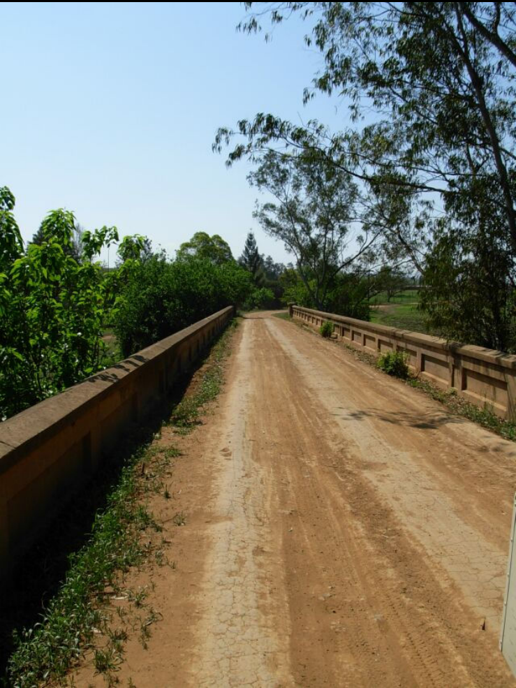
Figure 5: Southern view of bridge
