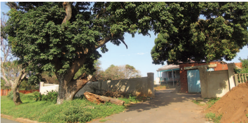
Fig. 18. The somewhat delapidated premises immediately opposite on 32 Moodie Street seen from Mackenzie Street.
