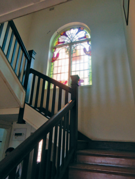
Fig.8. Wooden three-legged newel staircase.
