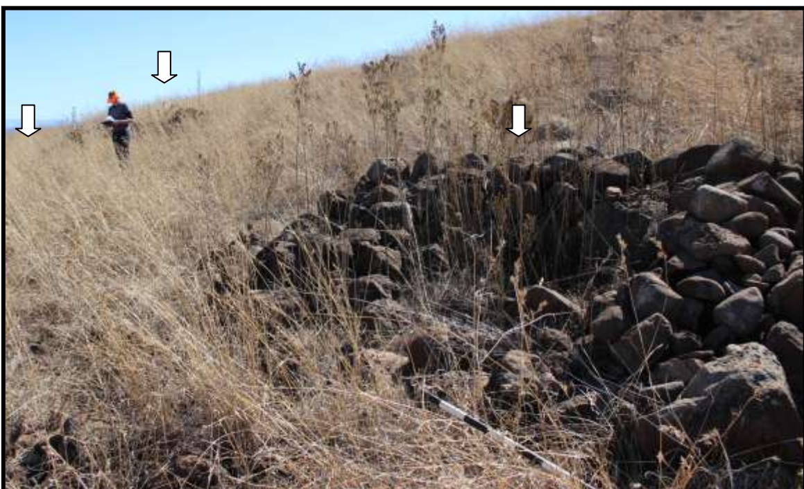
FIG. 11: STONE WALLING AT G25, G26, &G65
