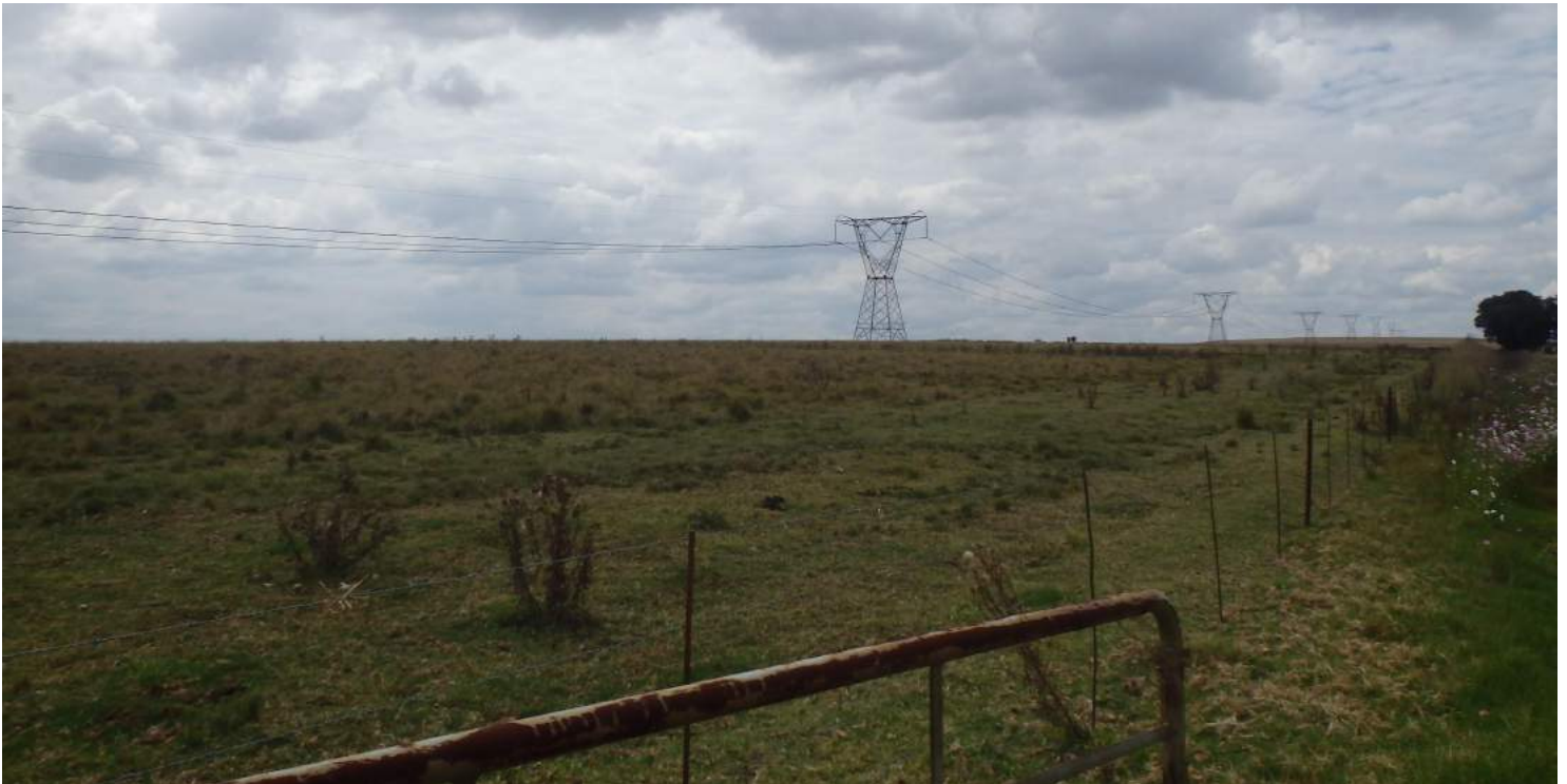
Figure 4.1: View of the 765kV overhead line running to Camden power station
