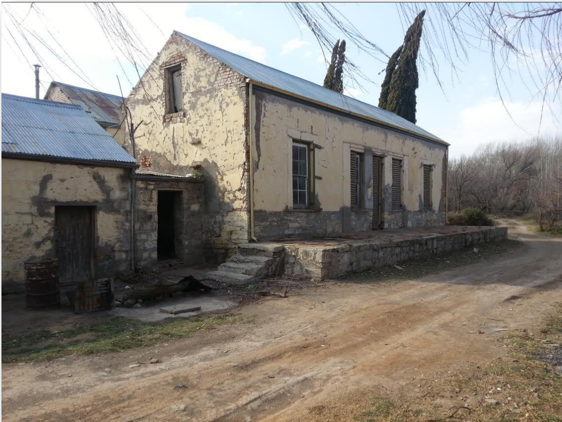
Figure 10 Un-occupied vernacular H-shaped house at Witteklip.
