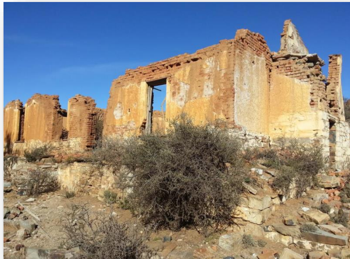
Figure 8 Ruins of a 19th century vernacular farm house at Klein Driefontein
