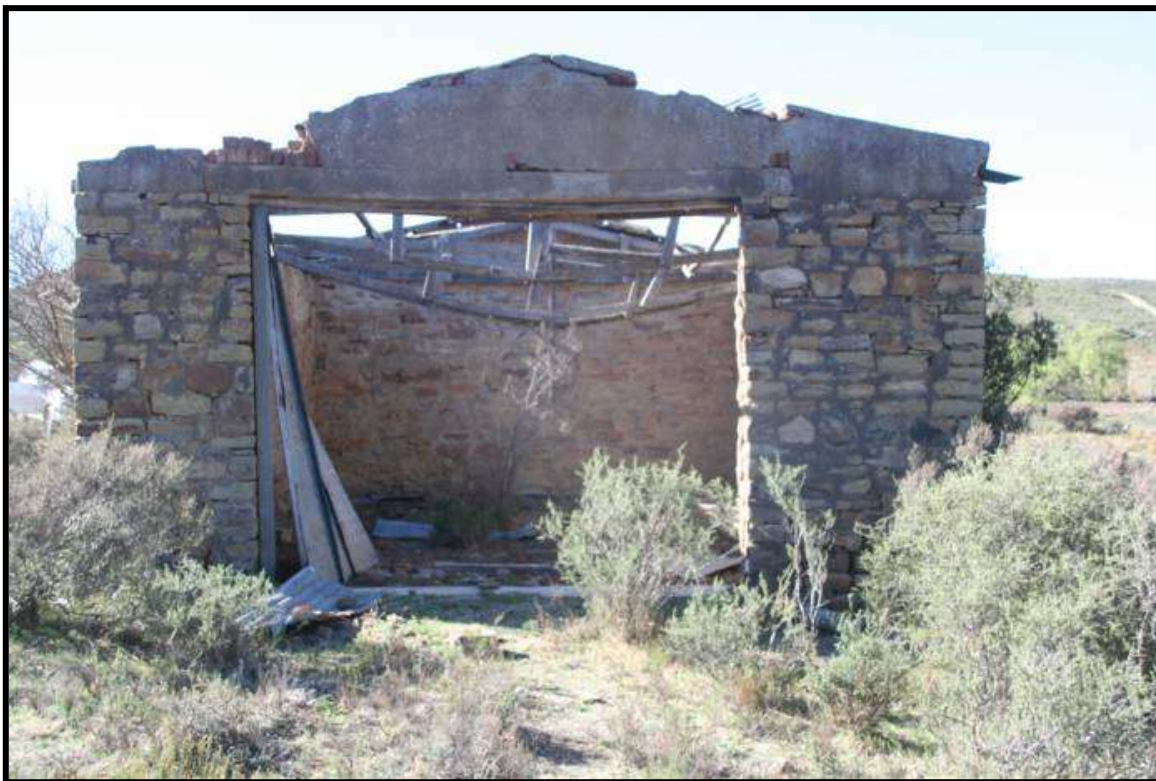
FIG. 11: SHED AT UMZ008
