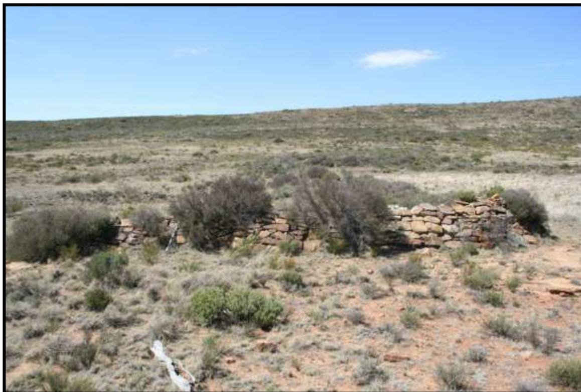
FIG. 16: SUPPORTING DAM WALL AT UMZ011
