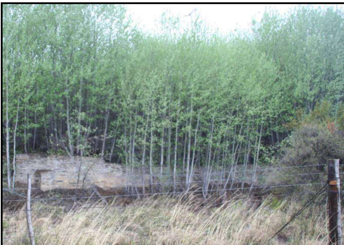
FIG. 9: WALLING AT UMZ002
