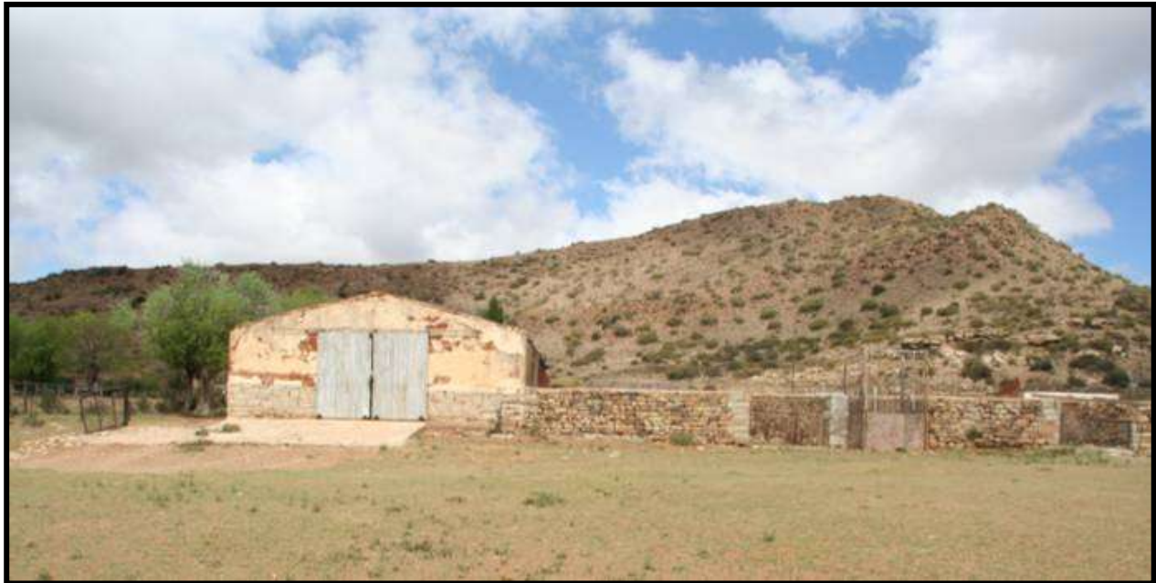
FIG. 36: SHED AND KRAAL WALLING AT WINTERHOEK
