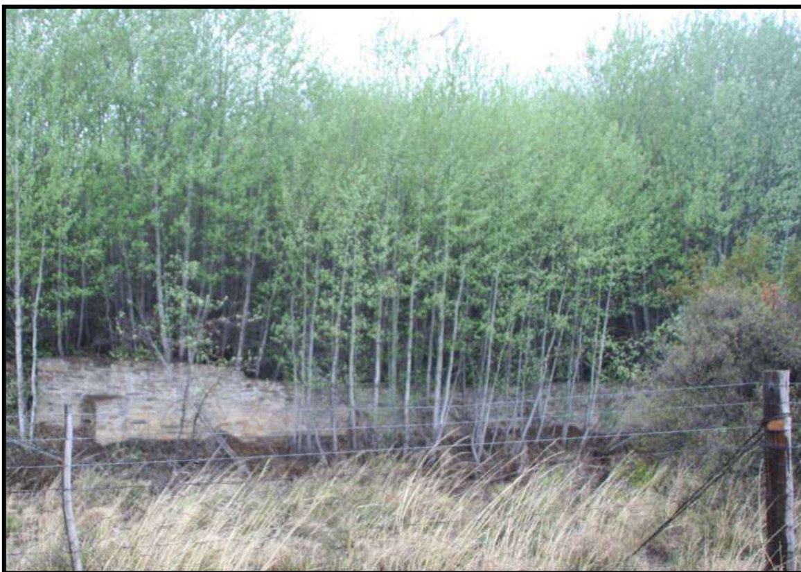
FIG. 10: WALLING AT UMZ002
