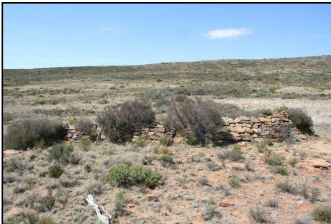
FIG. 22: SUPPORTING DAM WALL AT UMZ011
