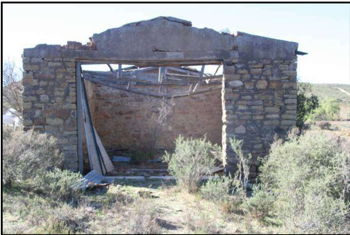
FIG. 16: SHED AT UMZ008
