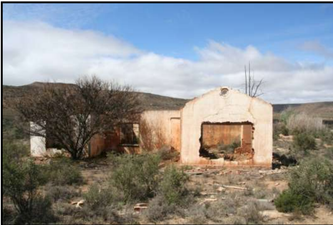
FIG. 45: FARM HOUSE DATING TO 1950
