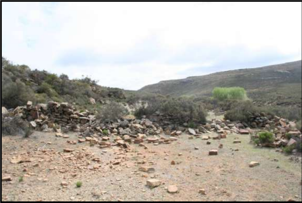
FIG. 32: STONE WALLING AT UMZ016
