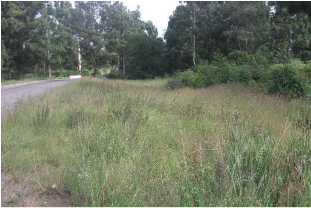
Figure 7: Pipeline route showing bridge crossing Mvubukazi River
