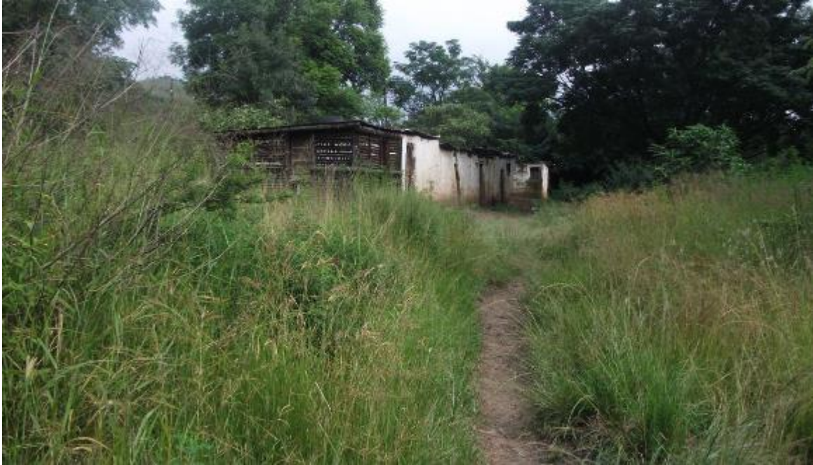
Figure 9: Buildings close to pipeline route
