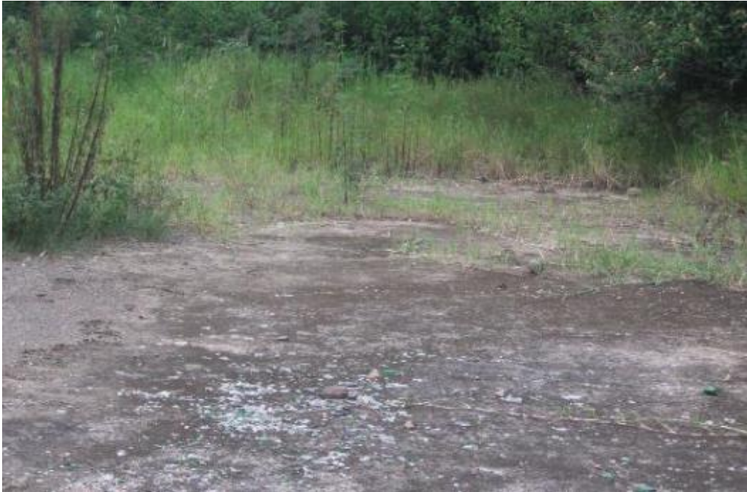
Figure 13: Remains of concrete floor
