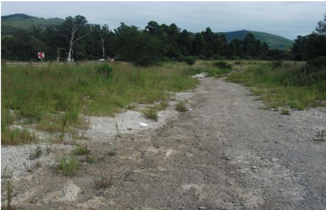
Figure 6: Looking northwards along pipeline route
