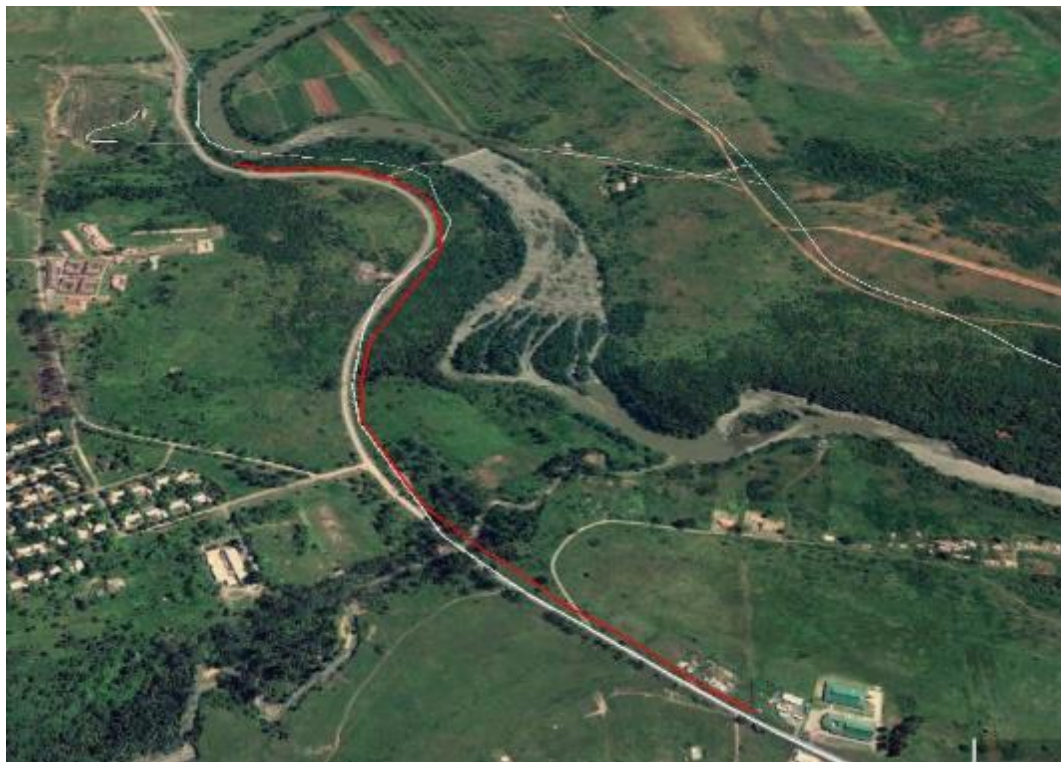
Figure 4: 2010 Google image showing buildings in south eastern corner
