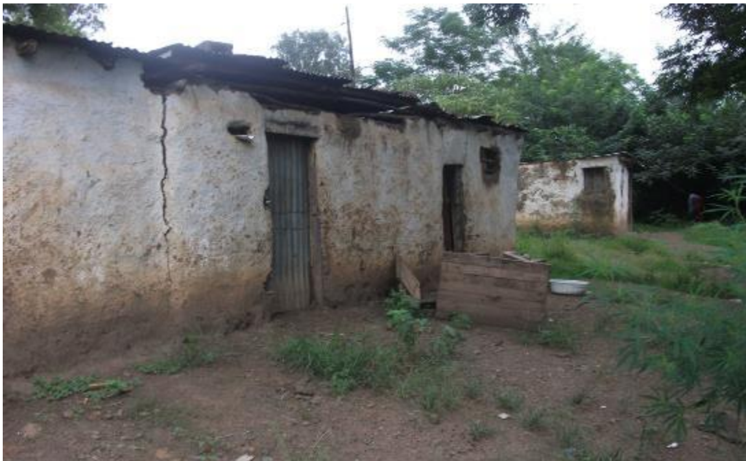
Figure 10: Section of building close to pipeline route
