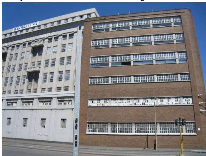
Fig 15: Sarnia road frontage of warehouse
