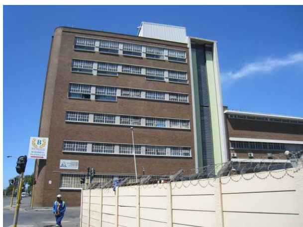
Fig 13: Northern façade of warehouse
