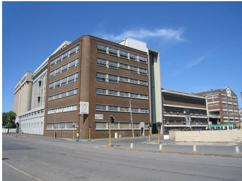
Fig 16: Corner warehouse on approach, and massing of site culminating in the verticality of the silo block
