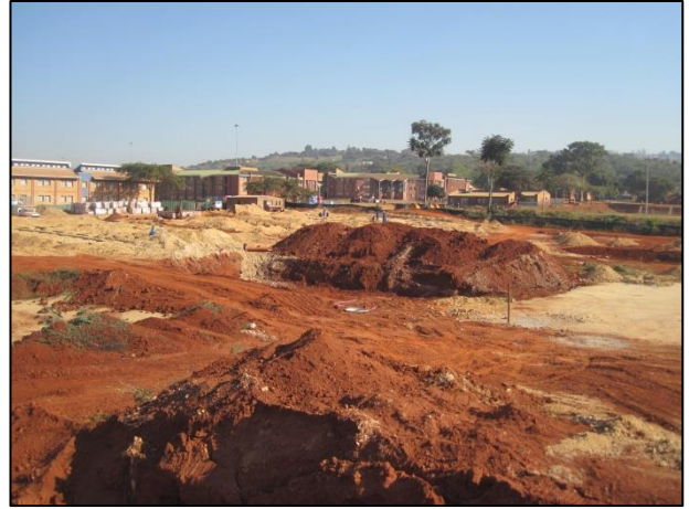
Figure 6: View of some of the earth-moving activities across the site.
