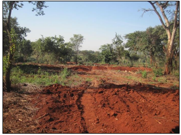
Figure 4: View of the recent bush clearing activities on the site.
