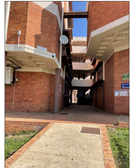
Figure 54H: Red brick & concrete features throughout.
