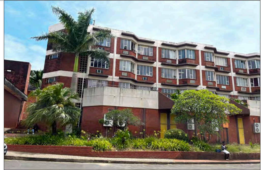
Figure 15A: Education building with face-brick, brise-soleil and concrete detailing. This building is surrounded by tropical vegetation, much like Brazilian Brutalism. (Authors own).
