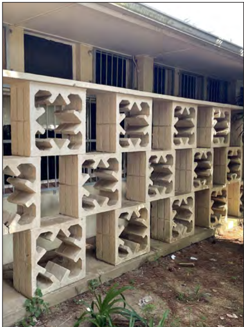
Figure 54C: Brise soleil and eaves on faculty bldg.
