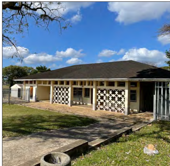
Figure 11B: An example of the patterned brise-soleil around the early academic buildings. (Authors own).
