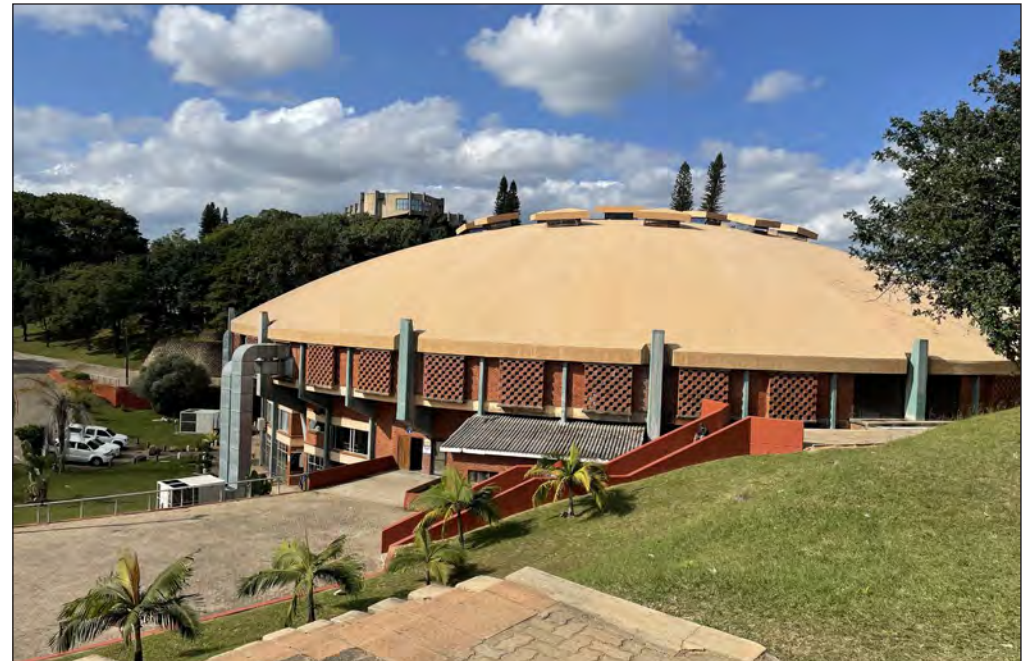
Figure 6H: The King Bhhekuzulu Hall is the ceremonial heart of the campus, and a noteworthy building.
