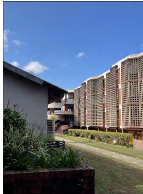
Figure 54G: More recent brises soleil.
