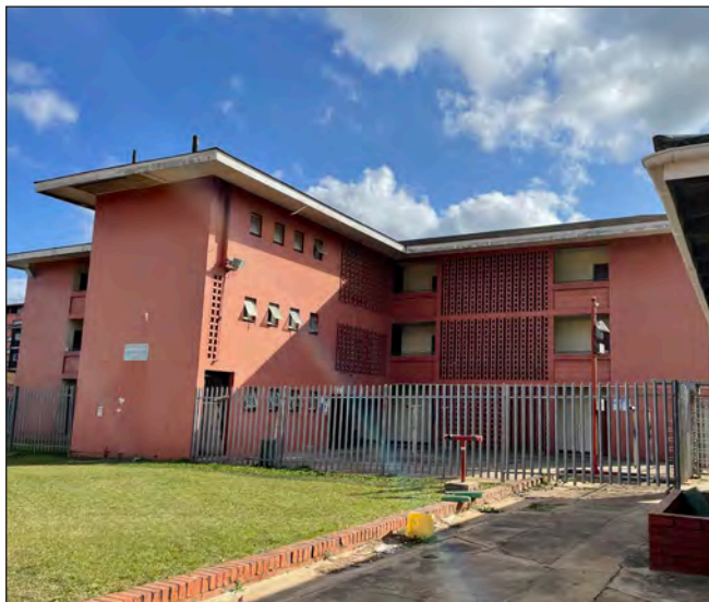
Figure 13B: Residential block with generic brise-soleil details and overhanging eaves. (Authors own).
