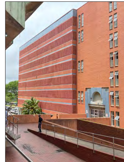
Figure 13D: Arts block with face-brick and generic brise-soleil type of this era. (Authors own).
