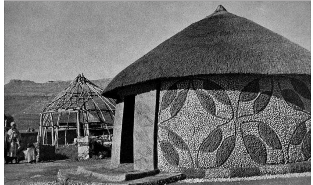
Figure 10: Taung hut with pebble mosaic decoration, Basutoland (James Walton, “South African Peasant Architecture: Southern Sotho Folk Building,” South African Architectural Record 34, no.1 [Jan. 1949], 2; 247.A.1.H[12b]).
