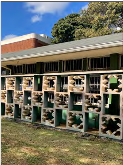
Figure 11A: An example of the brise-soleil around academic buildings. (Authors own).
