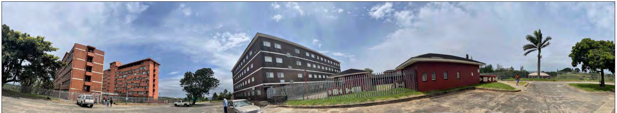
Figure 31B: The space between the “New York” and “Madiba” residences is unique because it frames two important vistas: the view over the Mangeza River valley to the north, and the view across the sports fields to the King Bheku
