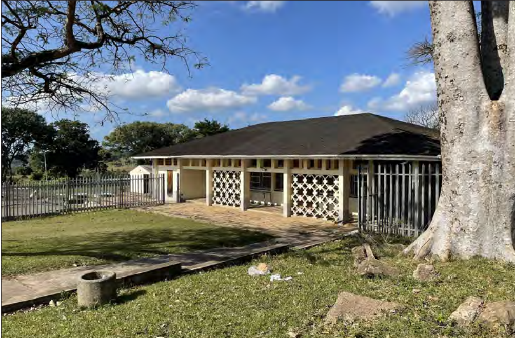
Figure 6C: One of the original academic buildings with an intact brise soleil.
