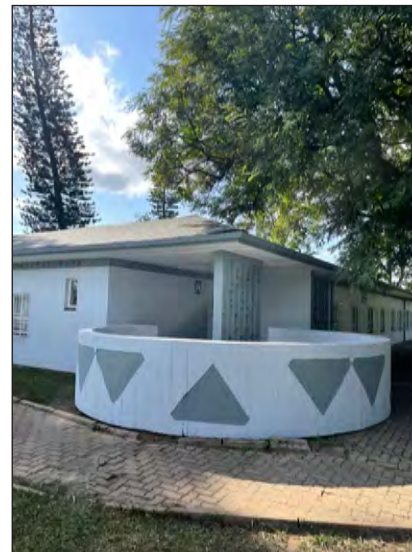
Figure 11C: Patterns of the brise-soleil, plaster detail and painting on early residential buildings. (Authors own).
