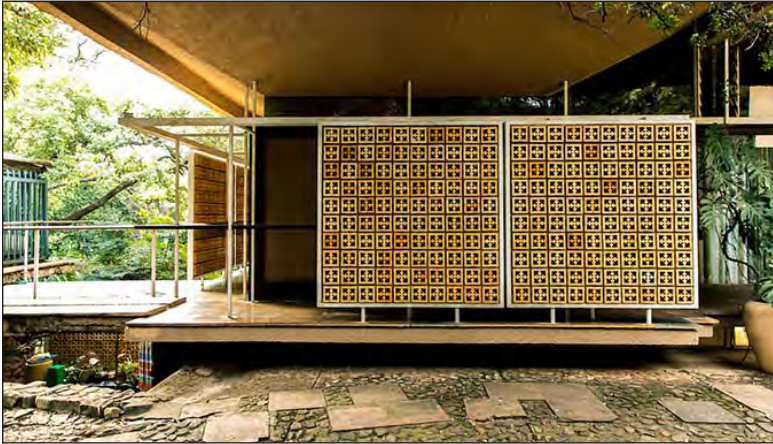
Figure 12A: House Van den Berg brise-soleil panels. (Image from Artefacts, taken by Cameron Forder, 2021).
