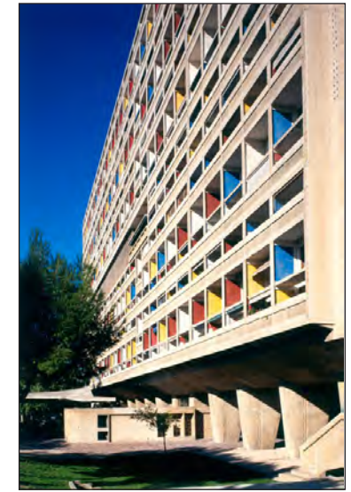
Figure 14B: Unité d'Habitation by architect Le Corbusier. (Brutalist buildings by Amy Frearson, 15 September 2014, Dezeen)
