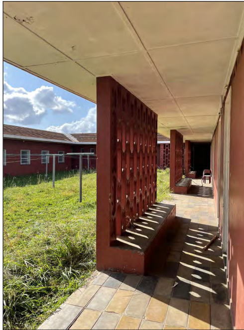
Figure 54B: Oversailing eaves and stoep area.
