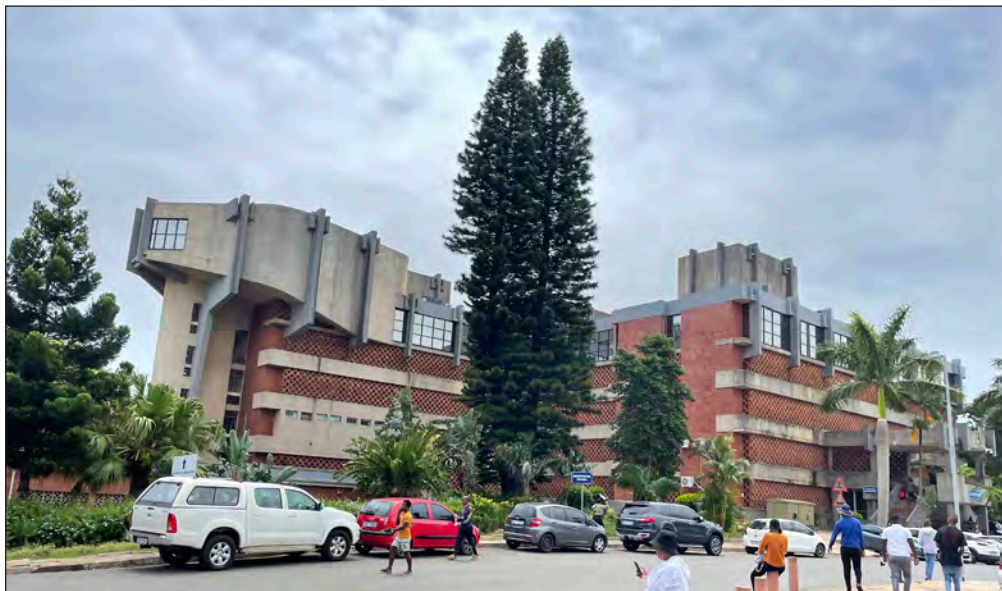
Figure 15B: Admin building with face-brick, brise-soleil and concrete detailing. This building is surrounded by tropical vegetation, much like Brazilian Brutalism. (Authors own).
