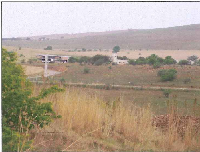
Fig 6: The Sterkfontein Caves Visitor Centre, as seen from Swartkrans, the view partially blocked by the signifier. It is raised on stilts to avoid seasonally waterlogged soils of the drainage line across which it is built. Its long double verandahs provide for shady areas for outdoor sitting and viewing. The complex includes a museum, restaurant, toilets and restroom, conference facilities, storage and a curio shop.
