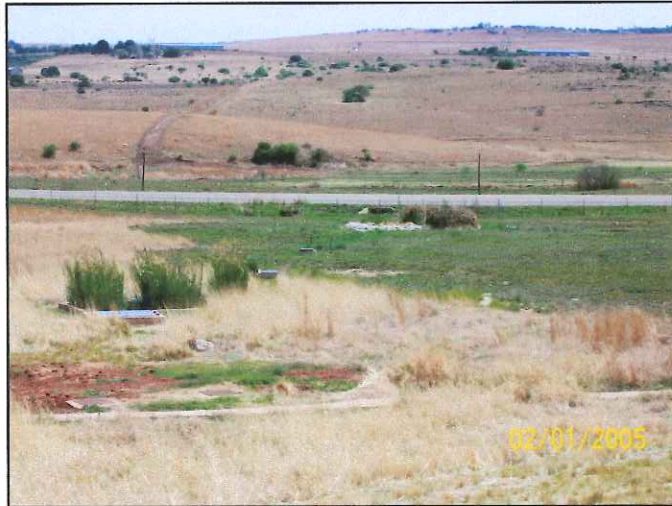
Fig 16: Reed beds damaged by fire. The reed beds are an integral part of the series of filtration ponds and repeated fires will destroy them Individual fire-breaks need to be cut around each installation.
