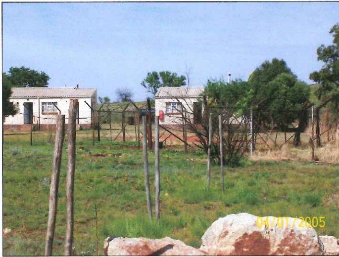
Fig 5: The old "Compound" complex, which houses the resident excavators working on the Sterkfontein Fossil Site and their families. Its management and upkeep are the responsibility of the University of the Witwatersrand. It requires a facelift and screening from public view, with the dual purpose of providing privacy for residents and to reduce visual impact.
