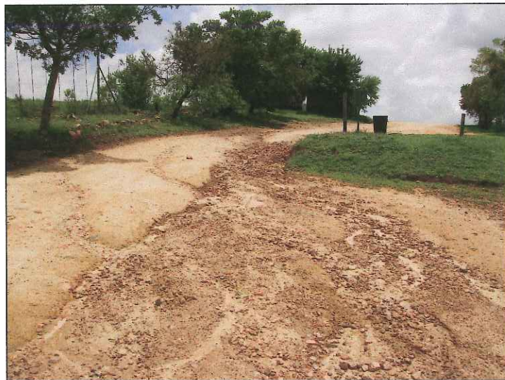
Fig 3: Erosion of the Wonder cave driveway, 2008
