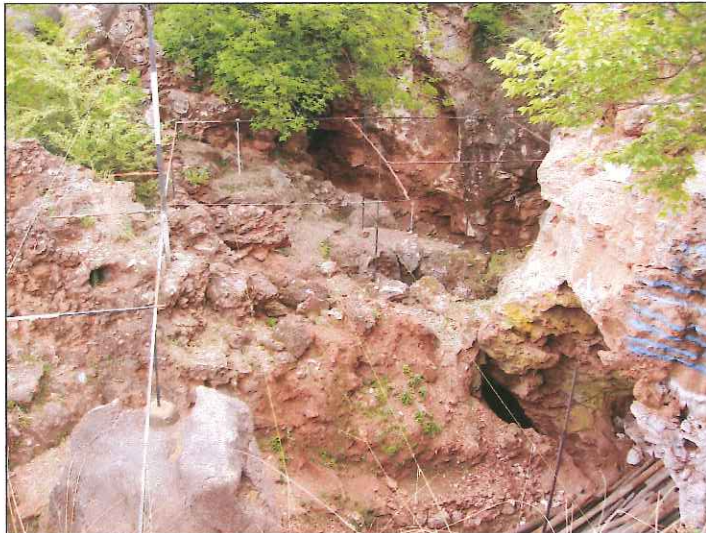
Fig 10: Hanging remnant area after removal of unstable breccia (replace picture)
