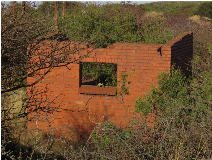
FIGURE 37: SECOND BUILDING ASSOCIATED WITH THE FIRST.
