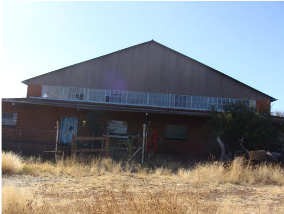
FIGURE 23: OLD RECREATION HALL CLOSE TO THE HOSTEL AREA.
