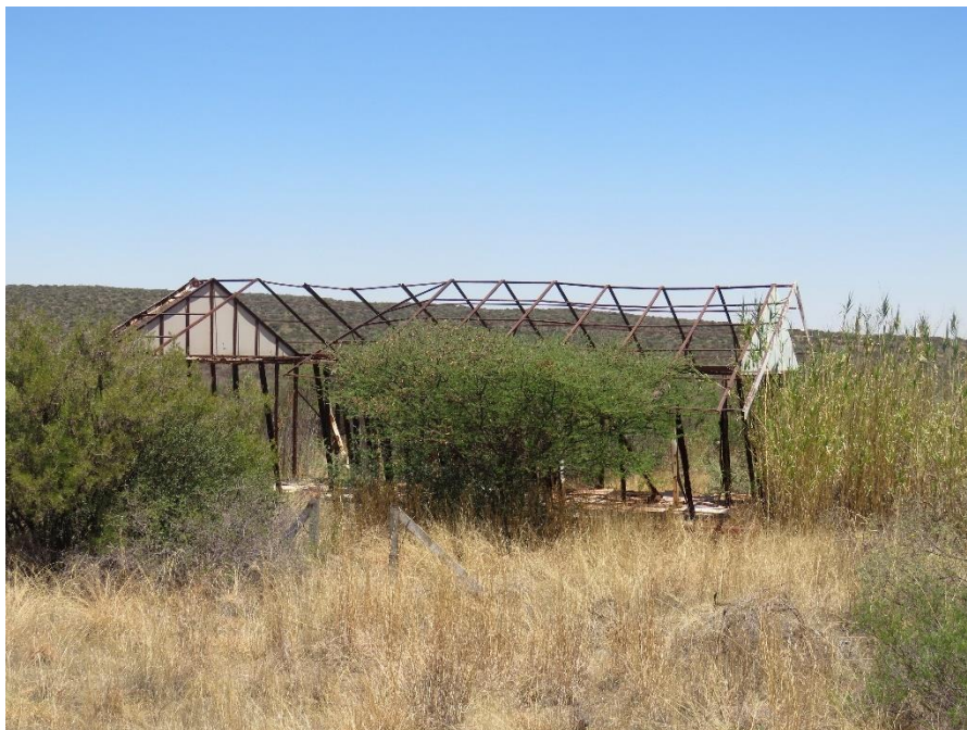
FIGURE 59: STEEL FRAME OF A RAILWAY BUILDING.
