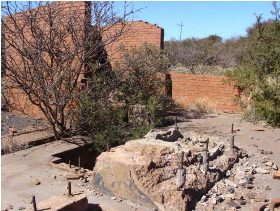
FIGURE 35: REMAINS OF AN INDUSTRIAL BUILDING IN THE MINING AREA.
