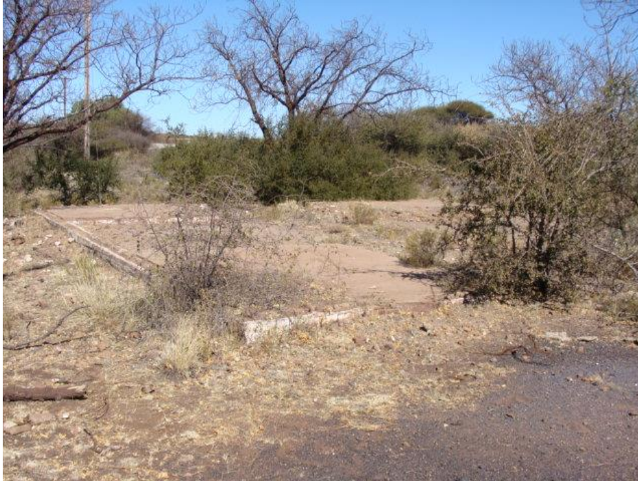
Figure 34: Foundation of a building less than 60 years old.
