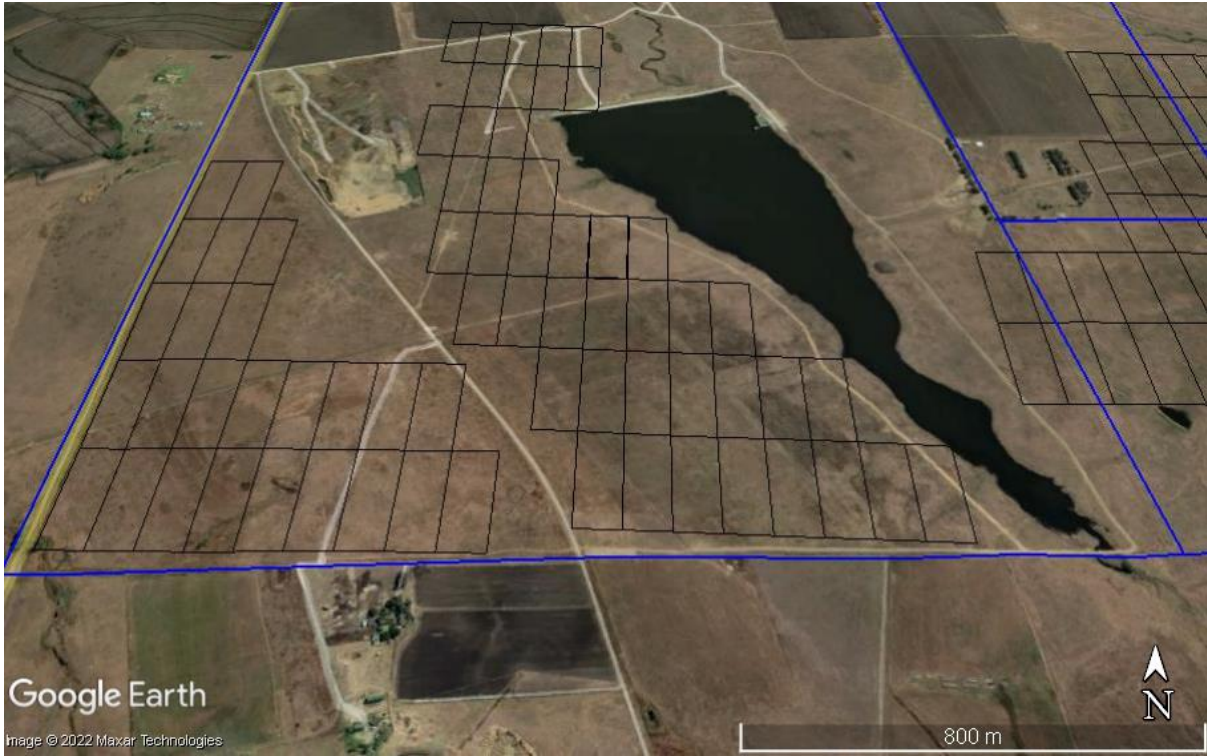
Fig 2: Vhuvhili Solar PVs – western area close-up.
