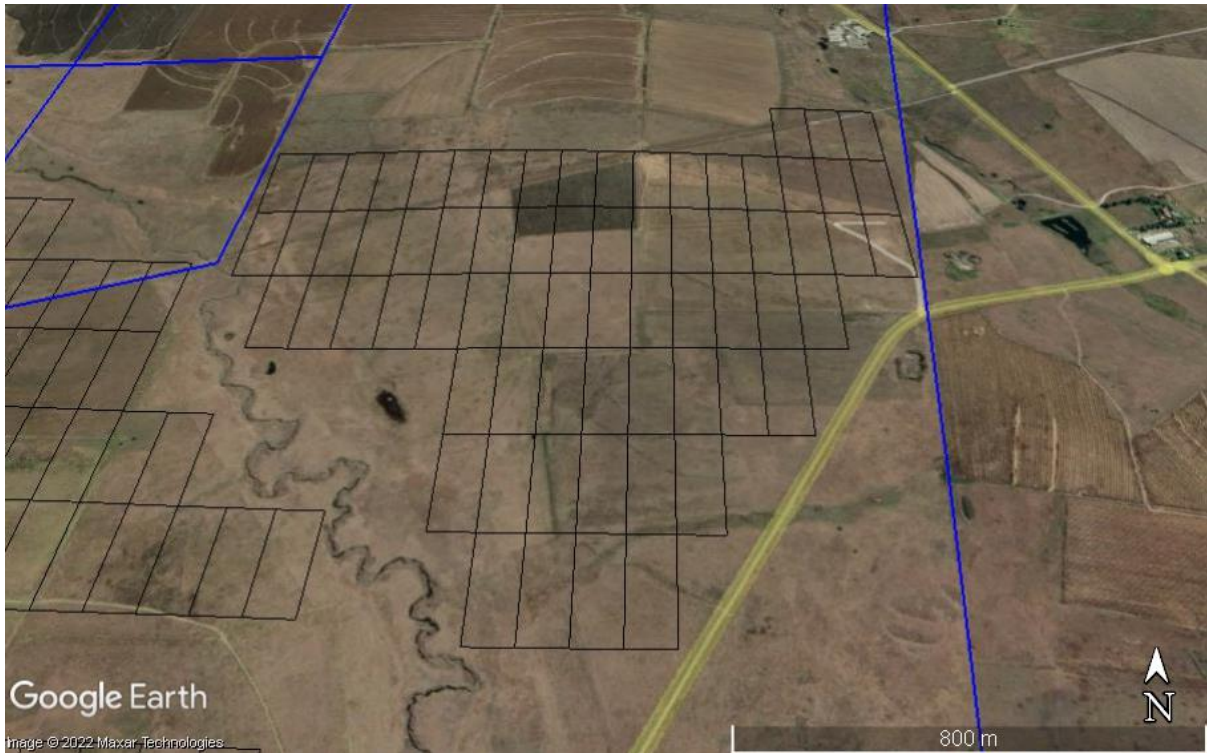
Fig 4: Vhuvhili Solar PVs – eastern area closeup.
