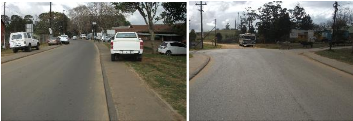
Figure 11: View of M30 to the south and to the north
