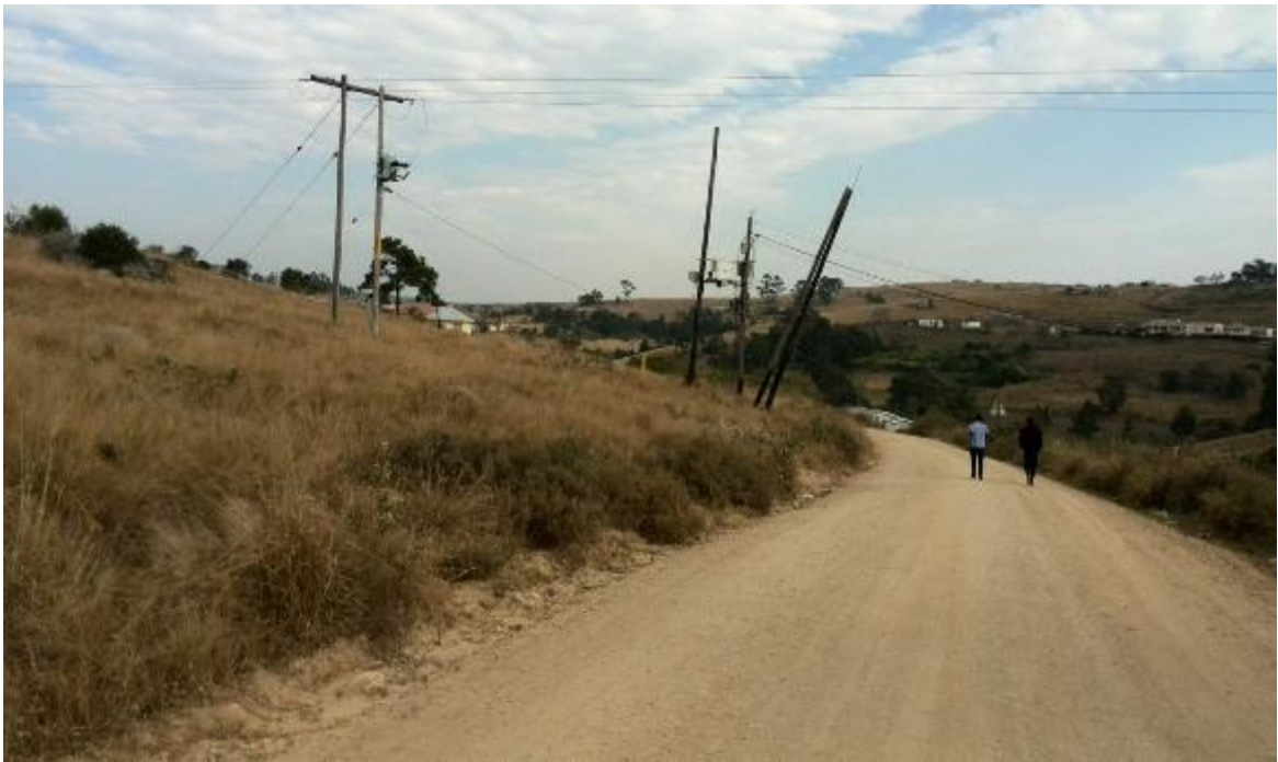
Figure 4: Existing infrastructure crossing D1095
