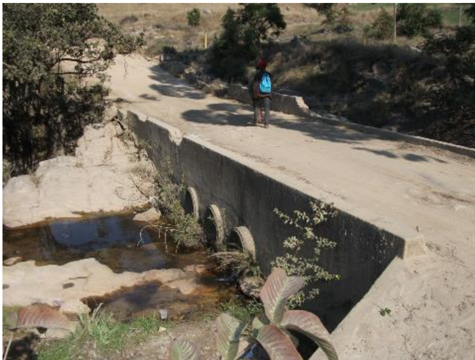
Figure 7: Concrete pipe / culvert 3
