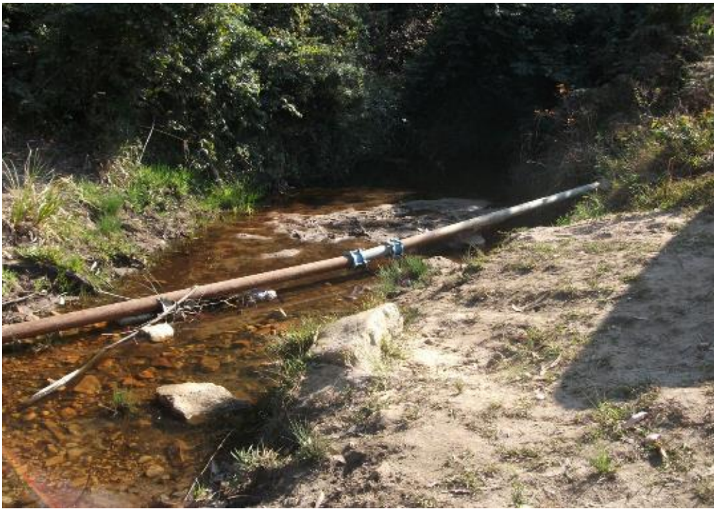
Figure 8: Water pipeline and thick vegetation in background
