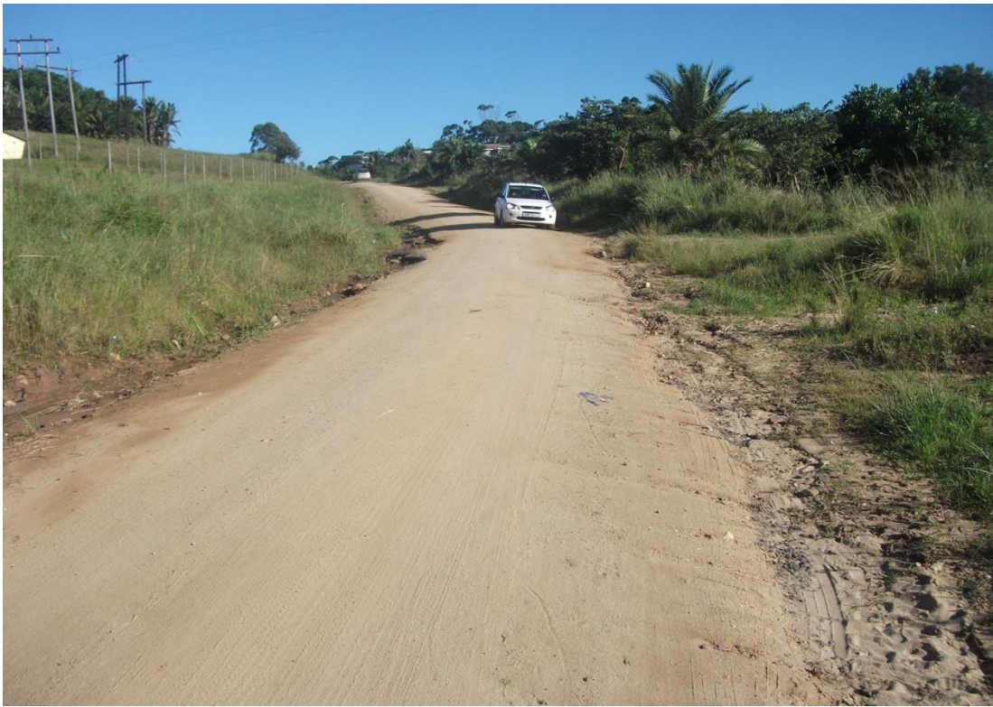
Figure 6: View northwards of condition of road
