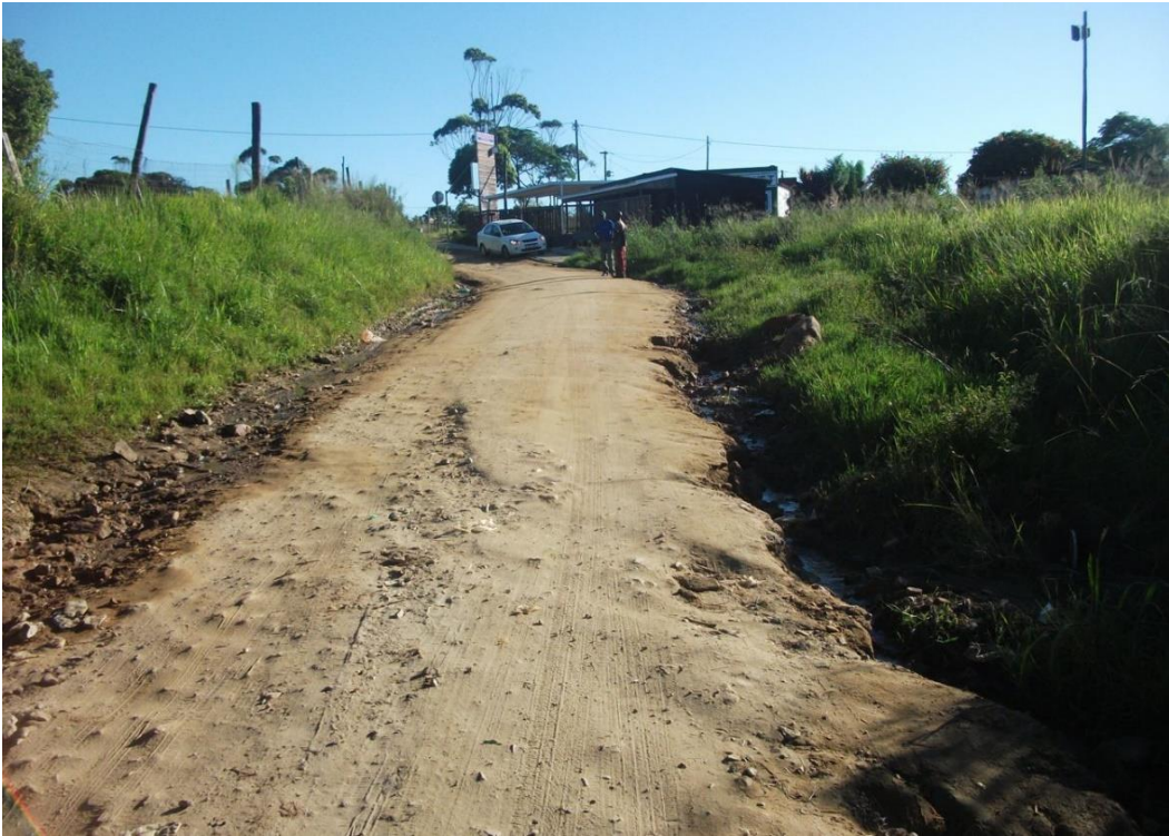
Figure 3: North-western start of road upgrade
