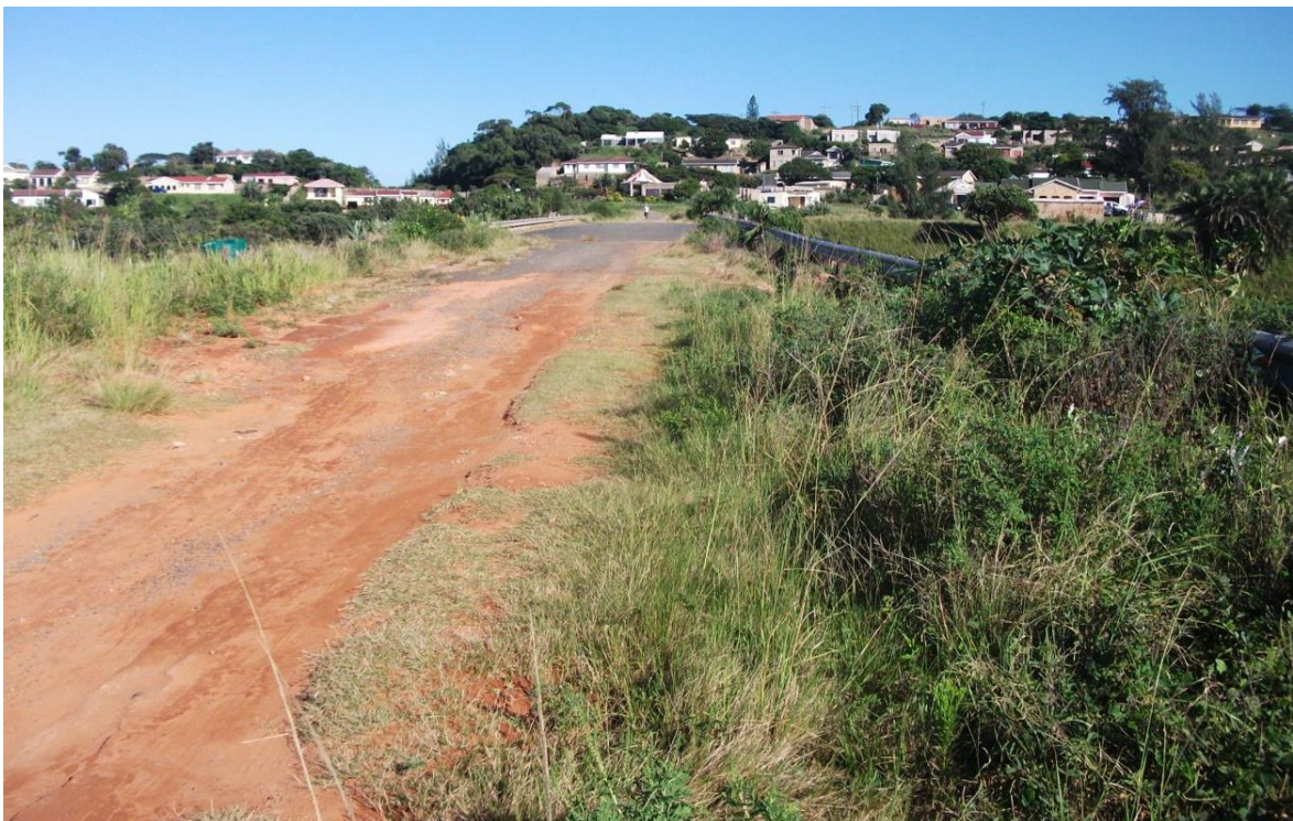
Figure 9: South-eastern end of road upgrade
