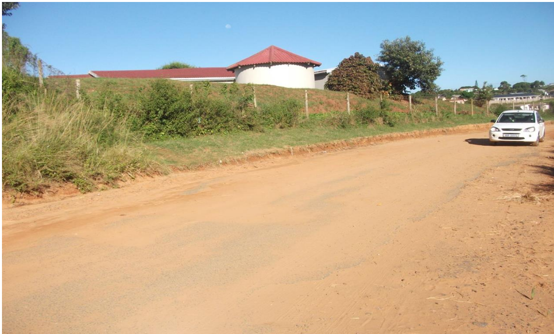
Figure 8: Section of tarred road and dwellings
