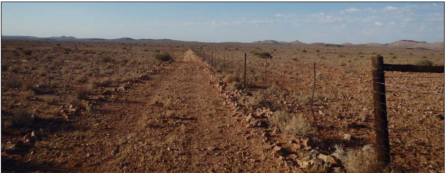
Figure 4.12: Pipeline route along fence
