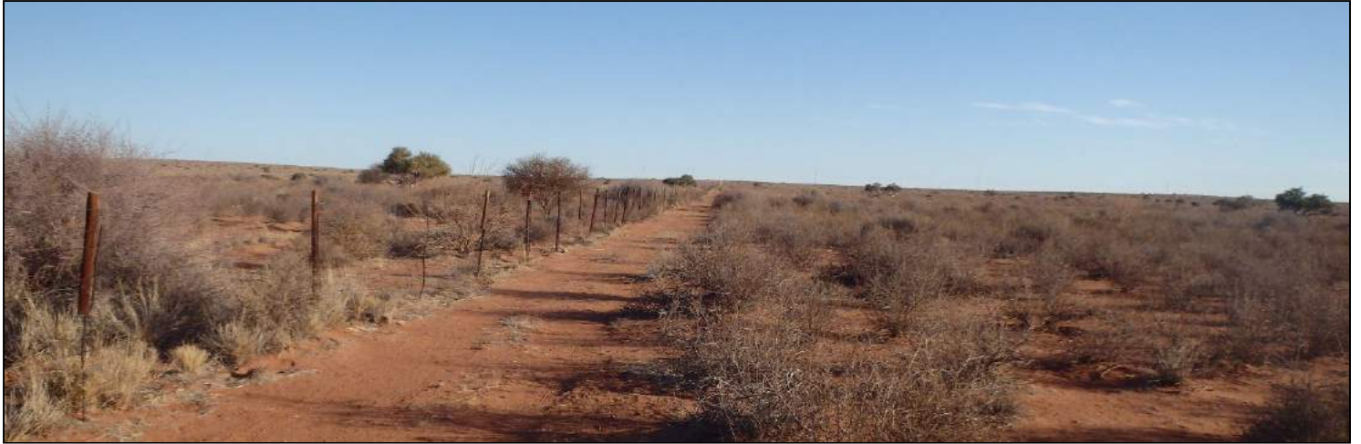
Figure 4.13: Pipeline route along fence
