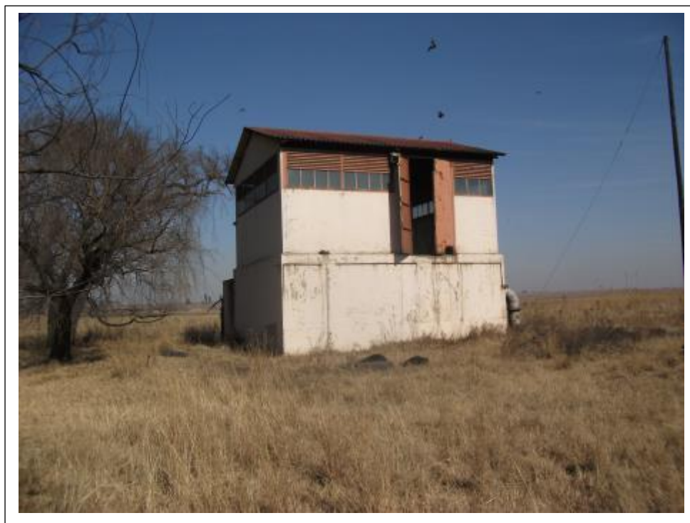
Figure 10- The former Douglas Colliers' pump station along the Olifants River.
