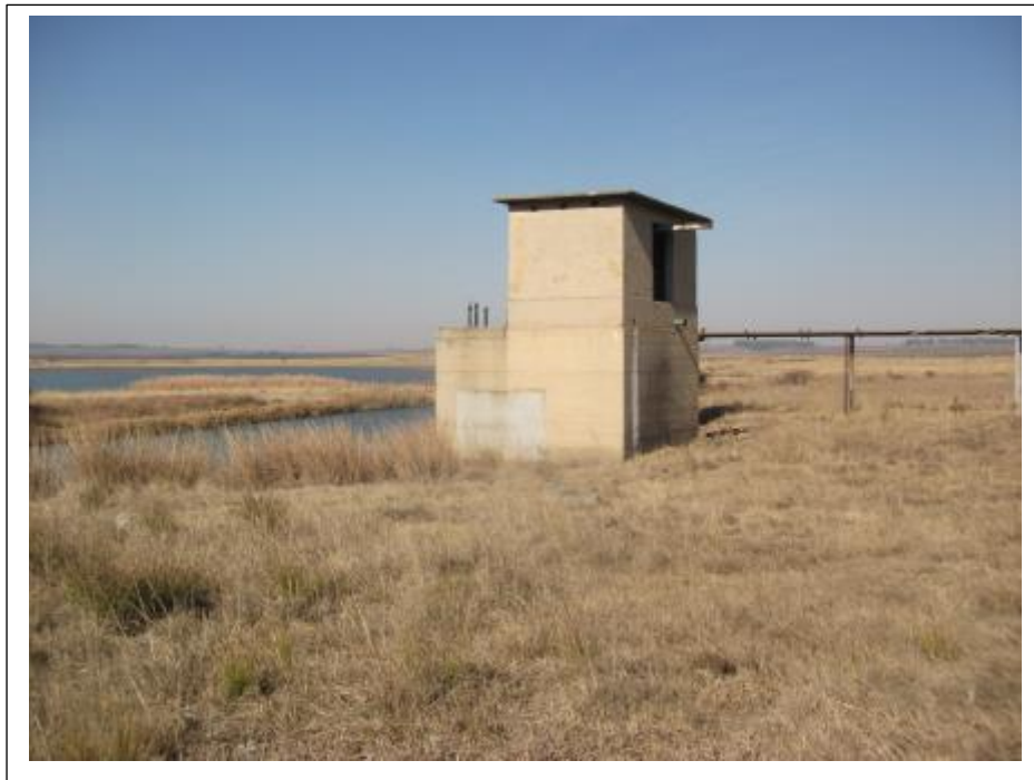
Figure 11- The pump station along the Olifants River which was used by the South African Railways.
