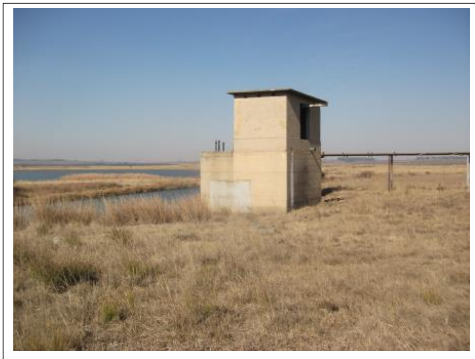
Figure 11- The pump station along the Olifants River which was used by the South African Railways (above).
