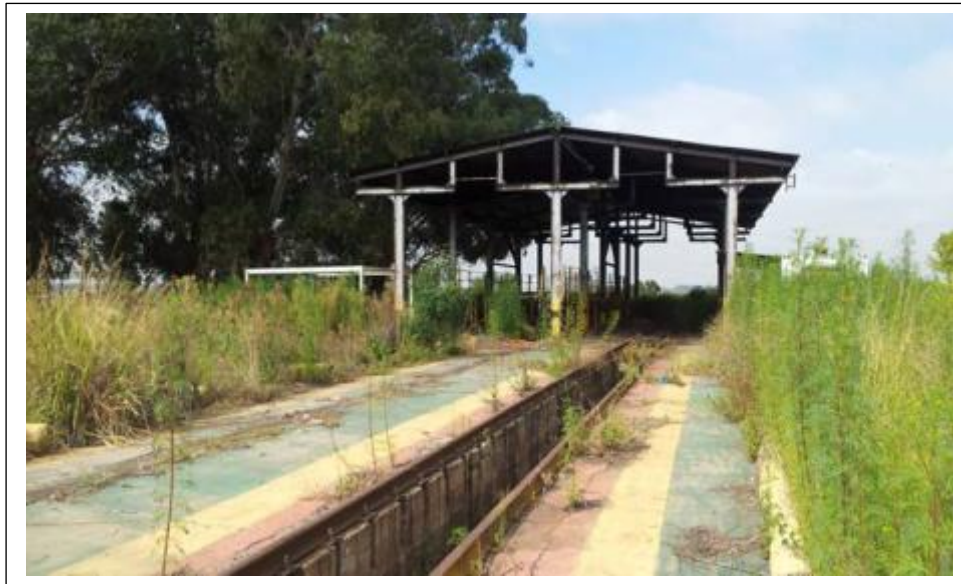
Figure 12- The rail way station along the railway line in close proximity of the Olifants River (Coetzee 2014) (above).
