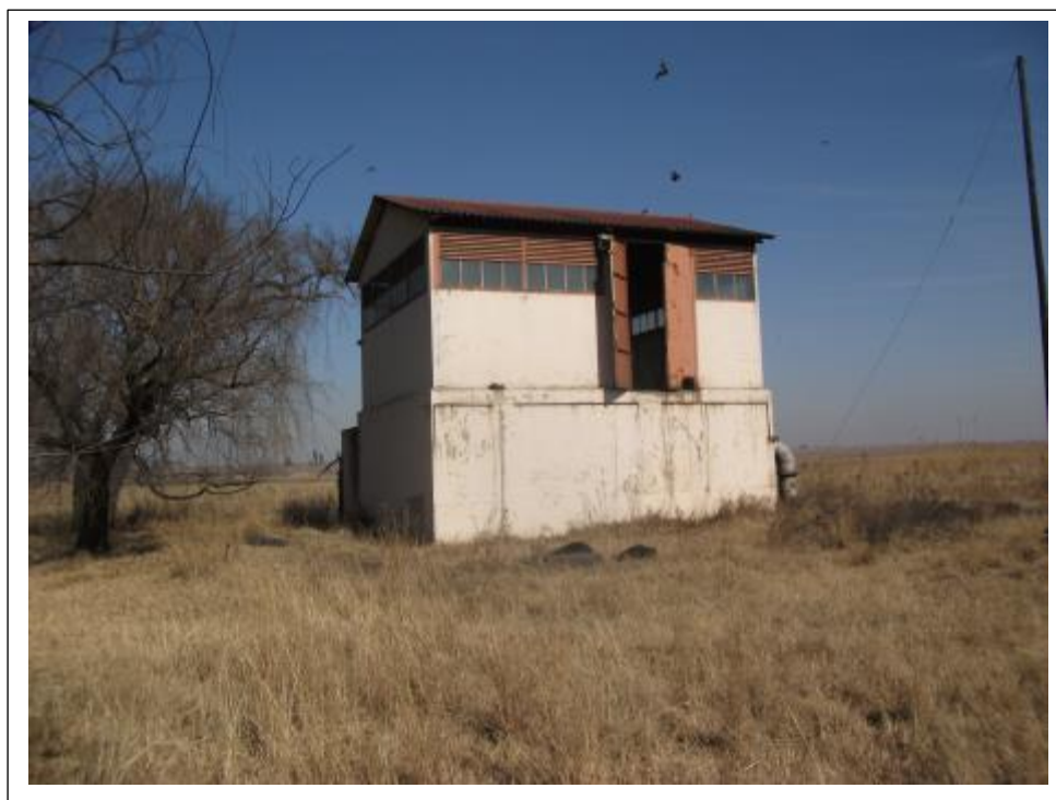
Figure 10- The former Douglas Colliers' pump station along the Olifants River (above).
